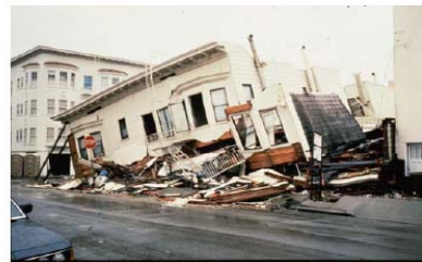
1994 Northridge Earthquake, Los Angeles (NIST)
