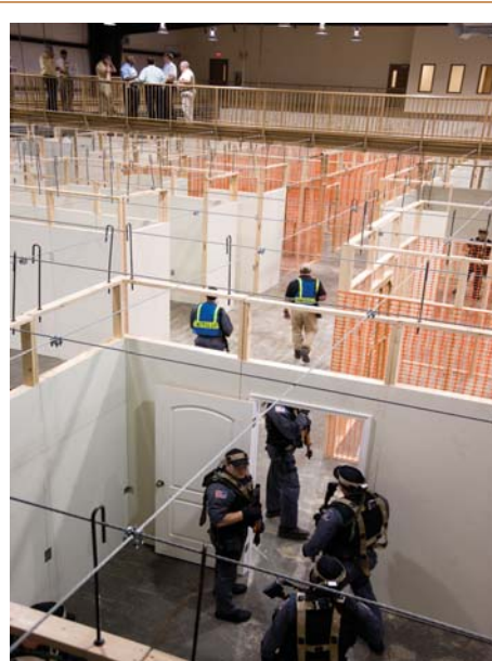
Oak Ridge Central Training Facility Shoot House
