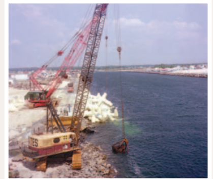
DOLOSSE PLACEMENT AT MANASQUAN INLET
