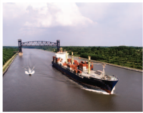
CHESAPEAKE & DELAWARE CANAL RECONSTRUCTION
