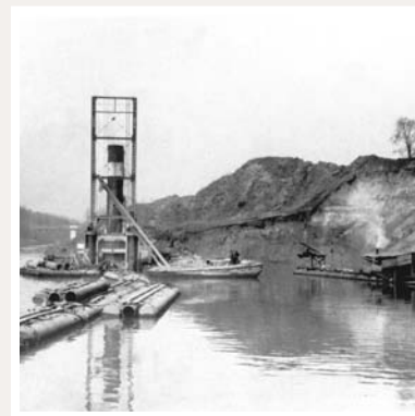
CHESAPEAKE & DELAWARE CANAL RECONSTRUCTION
