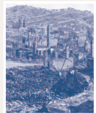
SAN FRANCISCO EARTHQUAKE
