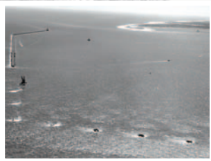
HARBOR OF REFUGE BREAKWATER
