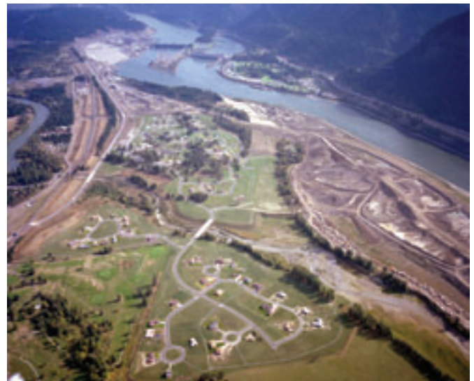
Relocation of the town of North Bonneville, downstream of the powerhouse construction.
