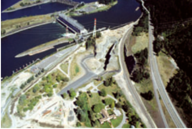
Progress on the excavation site for the navigation lock. The Union Pacific railroad tracks were relocated and the "stealth wall" built.
