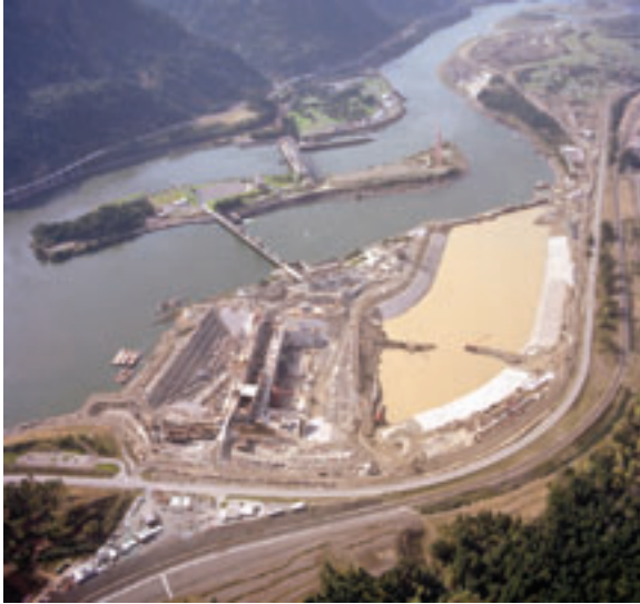
Concrete cut-off wall and the 40-acre excavation nicknamed the "bath tub"
