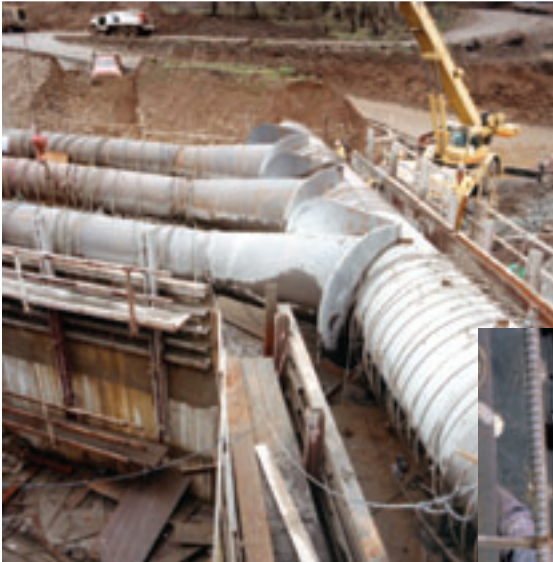
Laying the outlet pipes and constructing the first core of the dam
