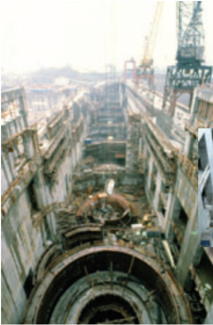
To complete the powerhouse in 54 months it took round-the-clock construction. Workers started at both ends and worked toward the center
