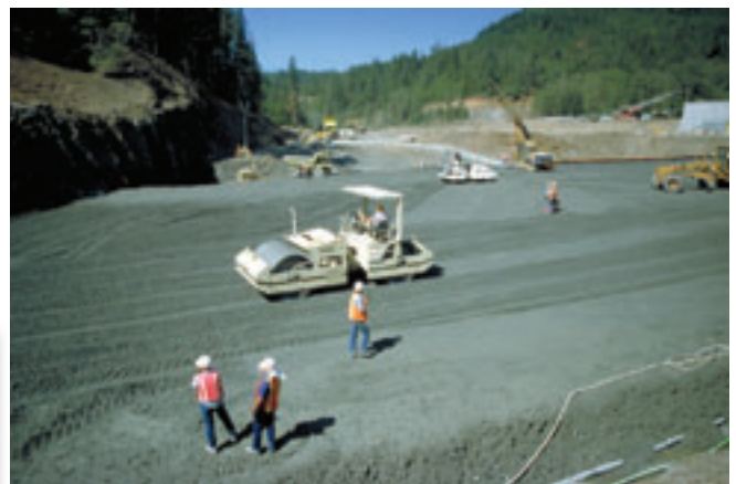
Roller compacted concrete (RCC) used on the surface of the structure
