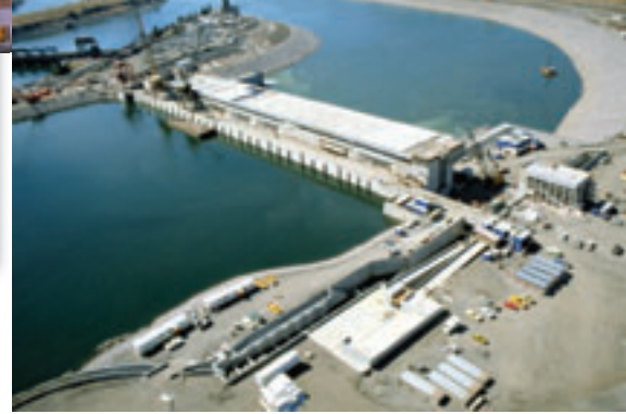
To complete the powerhouse in 54 months it took round-the-clock construction. Workers started at both ends and worked toward the center
