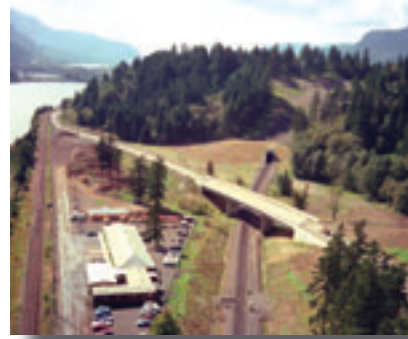
Relocated highway bridge and railroad underpass
