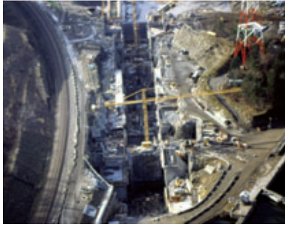
Progress on the excavation site for the navigation lock. The Union Pacific railroad tracks were relocated and the "stealth wall" built.
