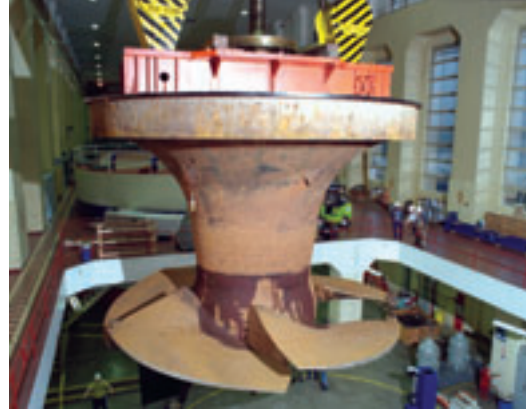
Work on the turbines in the First Powerhouse
