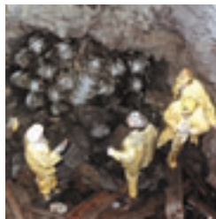
TBM BREAKING THROUGH THE SPIRIT LAKE TUNNEL
