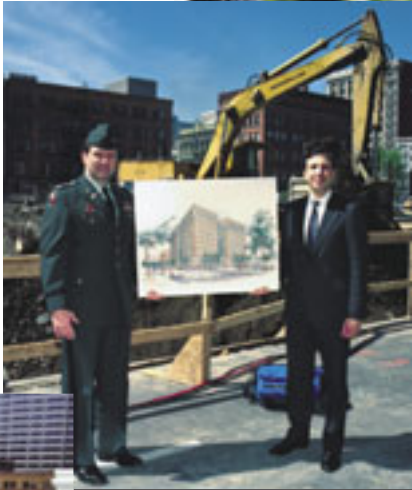
The construction of the Robert Duncan Plaza building, the new home for Portland District Corps of Engineers.
