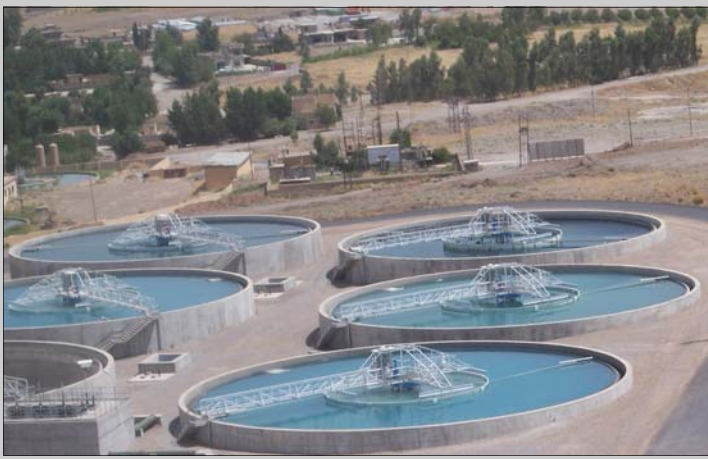
Erbil Water Treatment Plant, Erbil. Completed July 2006. Providing potable water to approx. 330,000 local residents.
