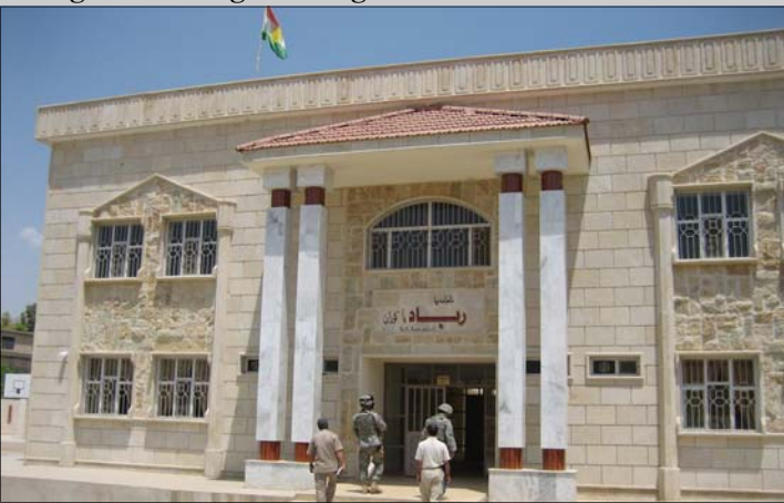
Sheile Primary School, Dahuk Province. The $416,000 model school new construction project serves 825 students.
