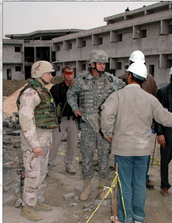
Rick Mers, left, project engineer, and Lt. Col. Dale Johnson, center, both with the U.S. Army Corps of Engineers, discuss progress on the prison with Iraqi engineers and construction company representatives during a January visit.
