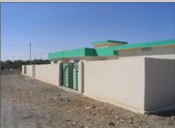
Ag Nimrud Agricultural Building – Ninewa Province – completed Nov. 4
