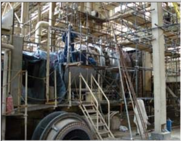
NGL/LPG Plant Repair – Basrah Province – estimated completion date — June 2007.
