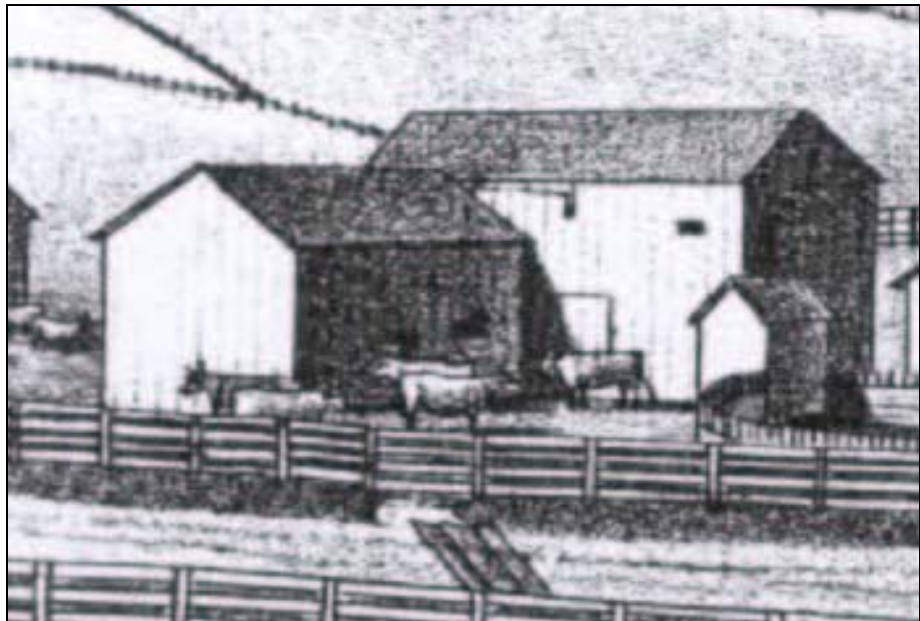
S. W. Elliott property, Rome Township, Bradford County. English barn with ell addition. From Craft 1878 history. Compare with site 117-WE-002 barn. (below)
