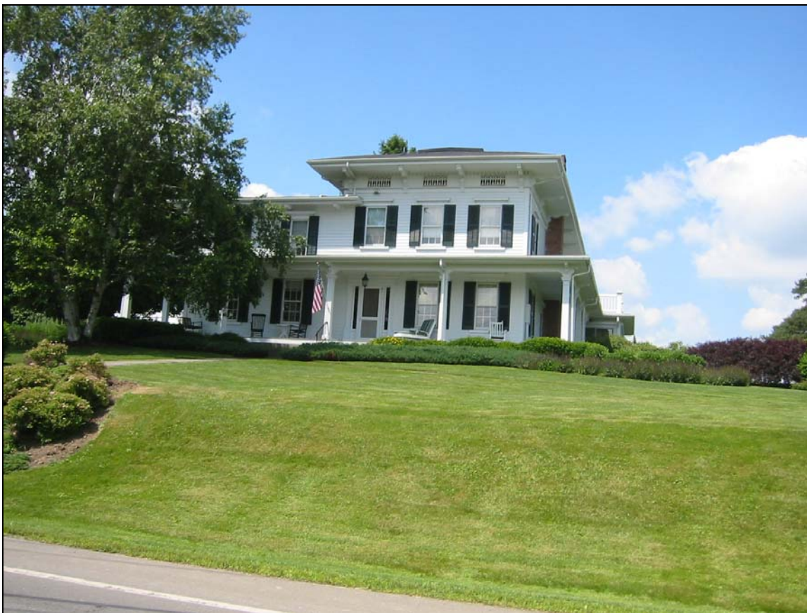
Bradford County Italianate house, site # 015-CA-002, Photo 4.
