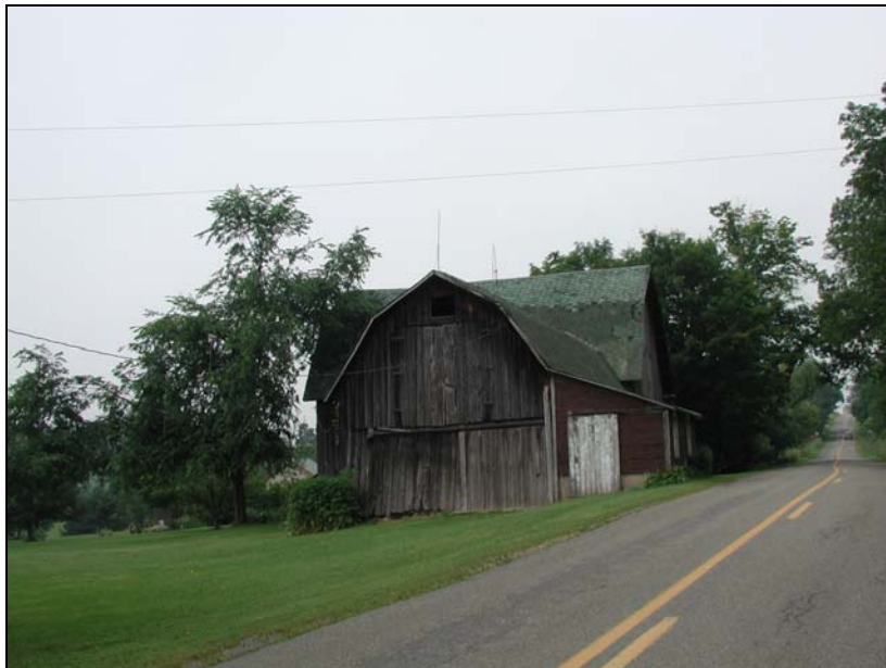
Bradford County – Ballard farm, gambrel roof English Barn with ell.
