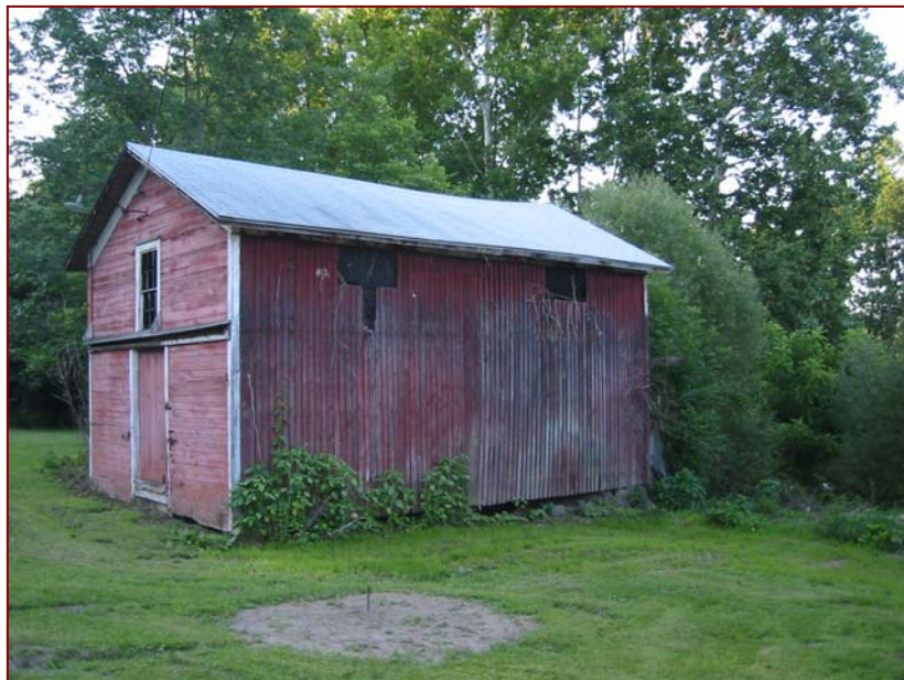
015-NT-001-05. Granary. Bradford County. This building has the trademarks of a granary: blank wall, raised off the ground, pass door in gable end, opening in second story gable end.
