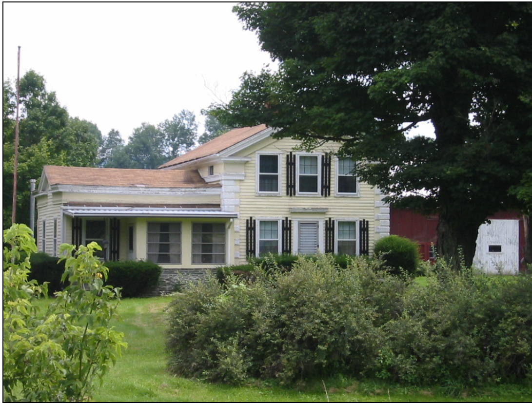
117-WE-001-01. Front of House. Tioga County, probably mid-19 th century. Upright and wing house, with eyebrow windows, wide fascia board, imitation quoins, and six over six-sash windows. This house represents the type nicely.
