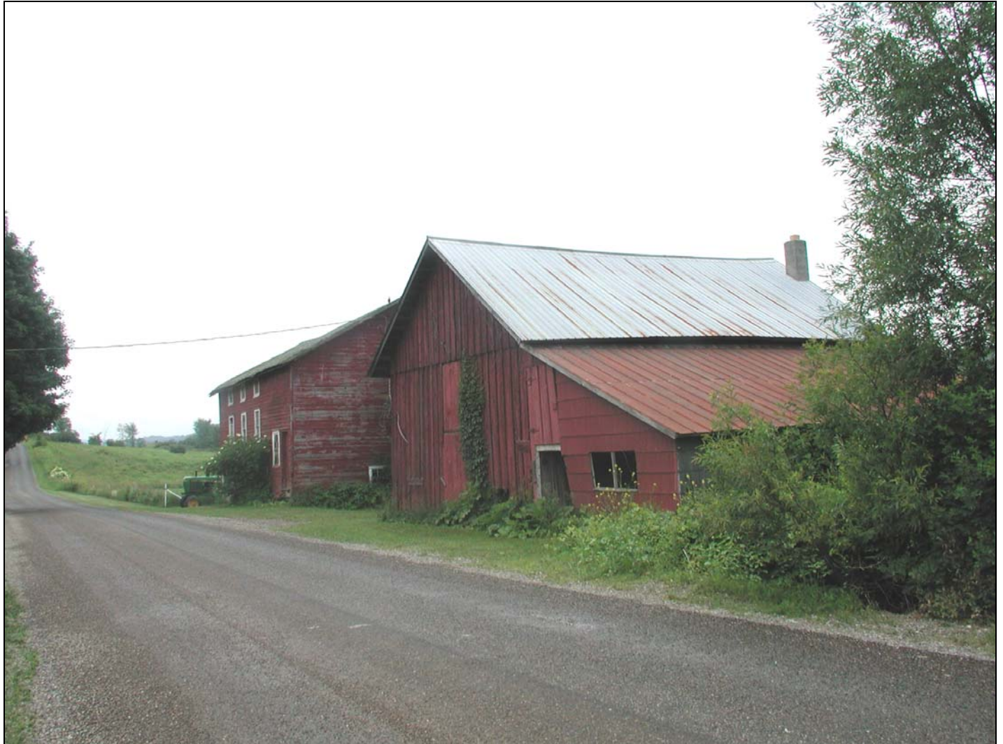
117-SU-001-05. Machine and poultry house from west. Tioga County. Machine shed is in the center.
