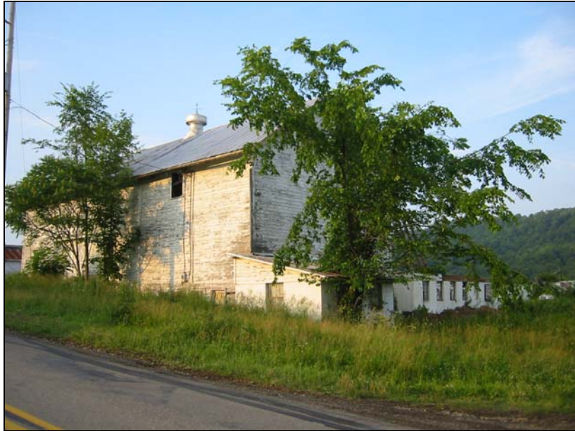
015-ST-001-01. Barn & Milk House. Bradford County. Basement barn.
