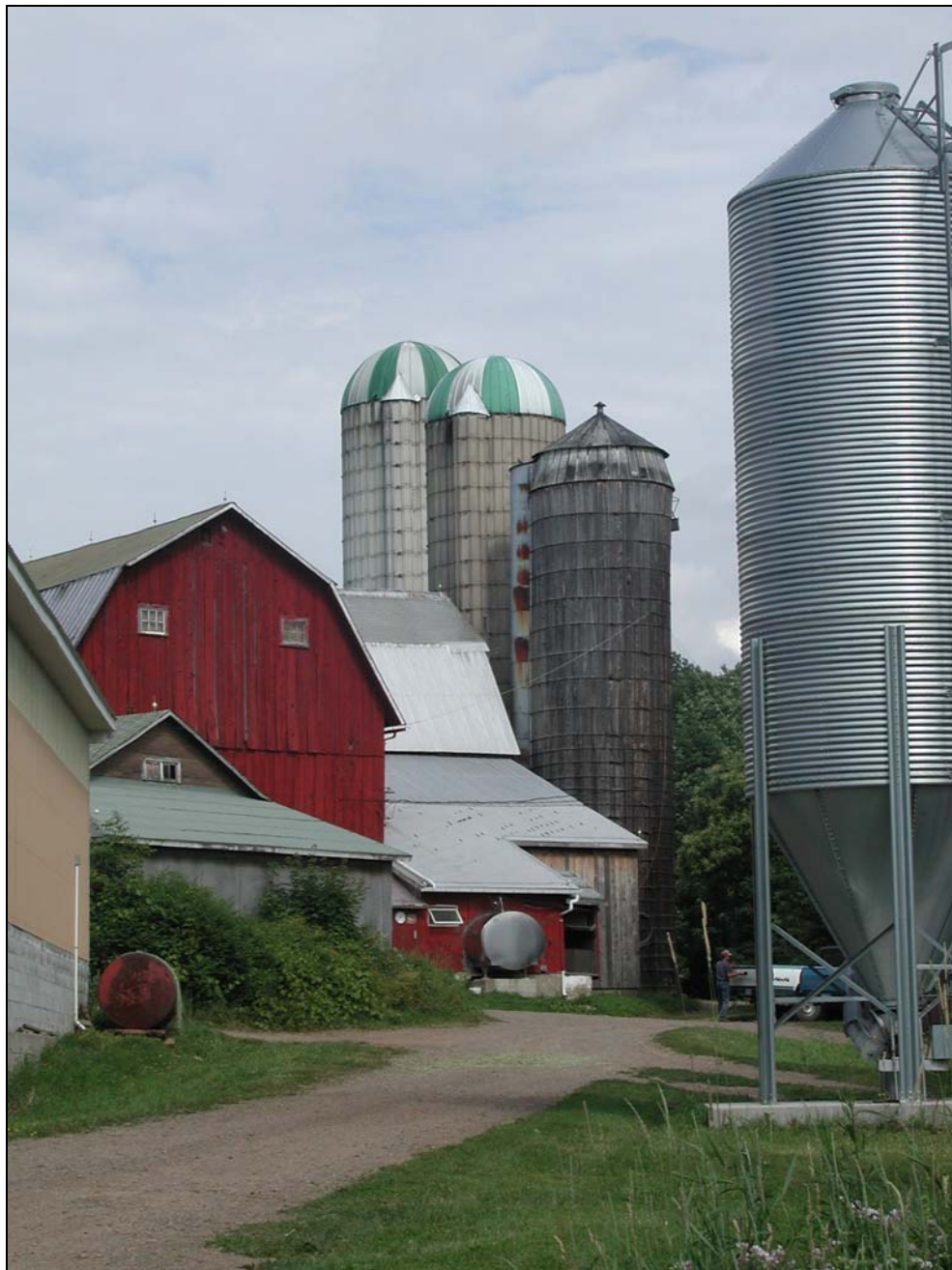
117-SU-004-11. Barns and silos. This Tioga County complex has a basement barn with several additions; a milk house, altered to accommodate a bulk tank; a wood stave silo probably from the 1920s, and two concrete stave silos.
