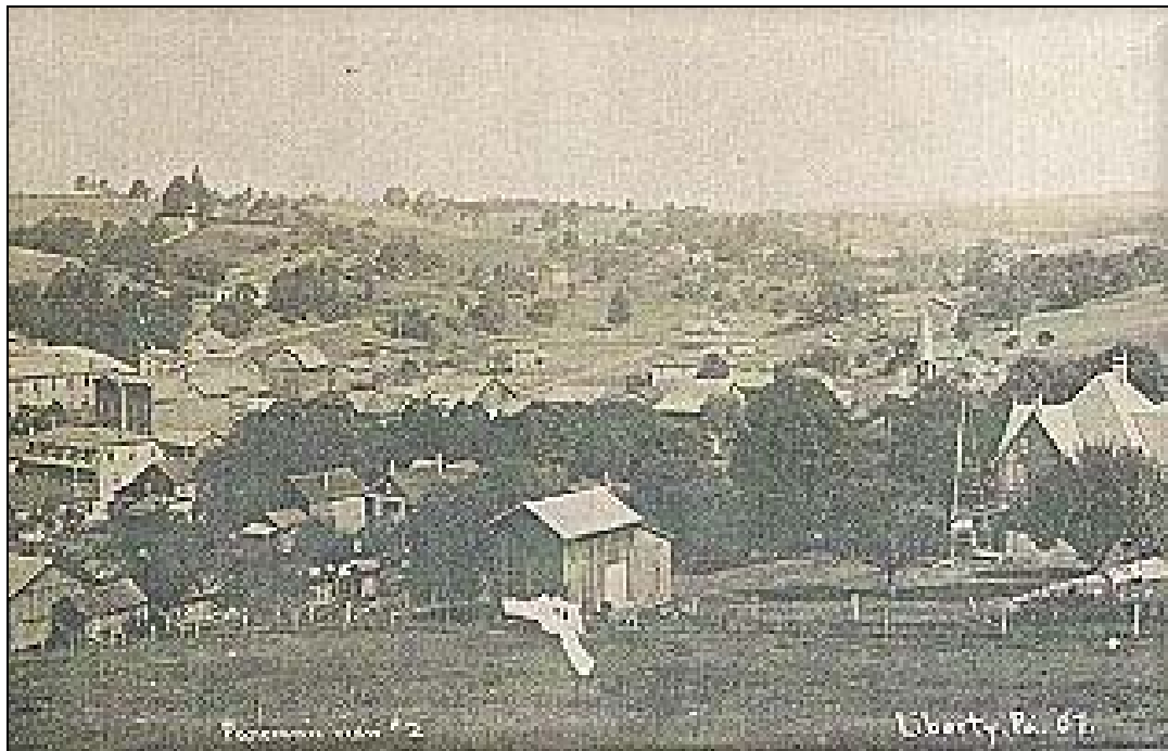
Liberty, PA, Tioga County, c 1907. Note worm and wire fencing; English barn in center foreground, with shed extension. From Tri Counties site.
