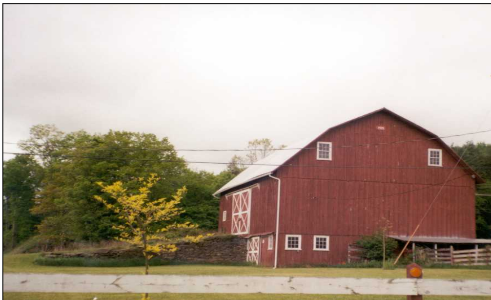
Basement Barn, northern Pennsylvania
