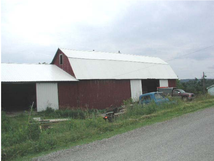
117-SU-006-01. Barn from road. Tioga County. A basement barn (right) with hay barn extension.
