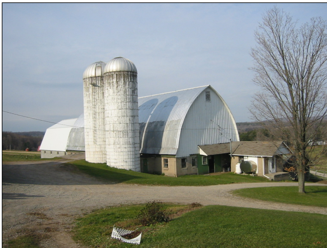
117-MO-002-19. Barn looking NW. This barn dates to 1954. Morris Township, Tioga County.
