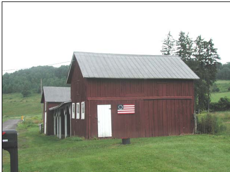
117-RU-002-09. Outbuildings, east side. This Tioga County site (below) shows a typical row of gable front outbuildings fronting immediately on the road. The near building has characteristics of a carriage or wagon shed; the far building probably housed poultry; while in between are open bays for implement storage and possibly also wood.
