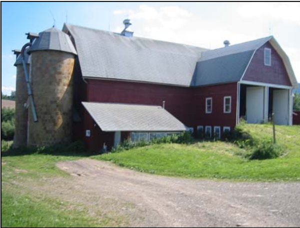
015-TR-04 Barn, Silos, Milk House, Bradford County
