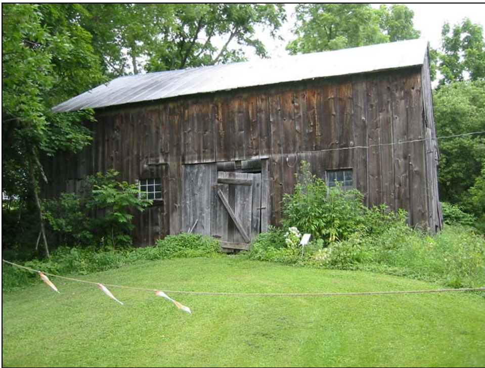
015-OR-001-114. Front of Barn. Bradford County. English barn. Dating before 1878.
