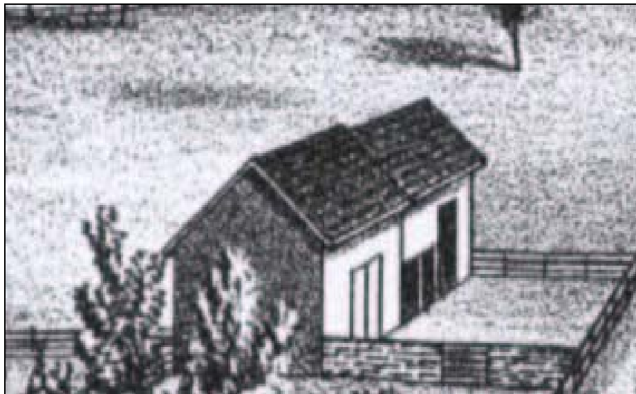
Ezra Ruty property, North Towanda Township, Bradford County, English barn with gable-end addition. From Craft 1878 history.
