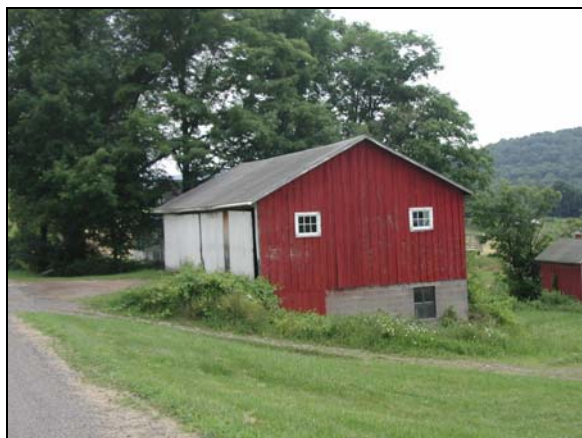
117-SU-005. Concrete block, board and batten garage, probably using recycled materials. Tioga County.
