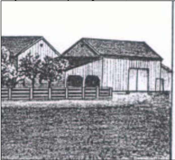
Joseph McKinney property, Athens Township, Bradford County. English barn with shed additions on gable ends. From Craft 1878 history.
