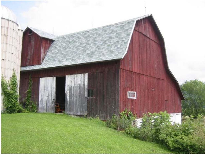
117-LA-001-06 Side and front of dairy barn. Basement barn, Tioga County.
