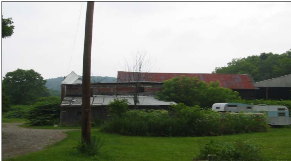
015-LI-001-02. Blacksmith Shop, Bradford County.
