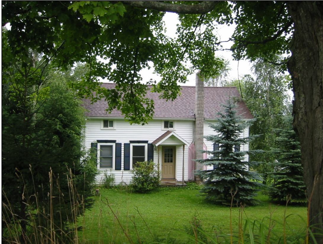
105-WB-001-04. Front of House (looking E). A Potter County house. While this house possesses little in the way of ornament, the proportions and eyebrow windows are faint echoes of Yankee/Yorker aesthetic vocabulary.
