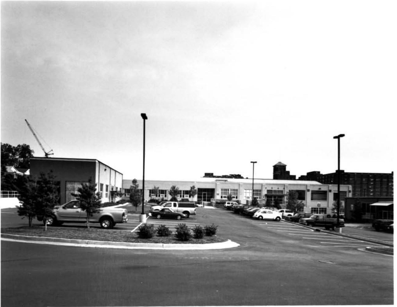
EMPIRE MANUFACTURING COMPANY BUILDING ATLANTA, FULTON COUNTY, GEORGIA PHOTOGRAPH 6 OF 15
