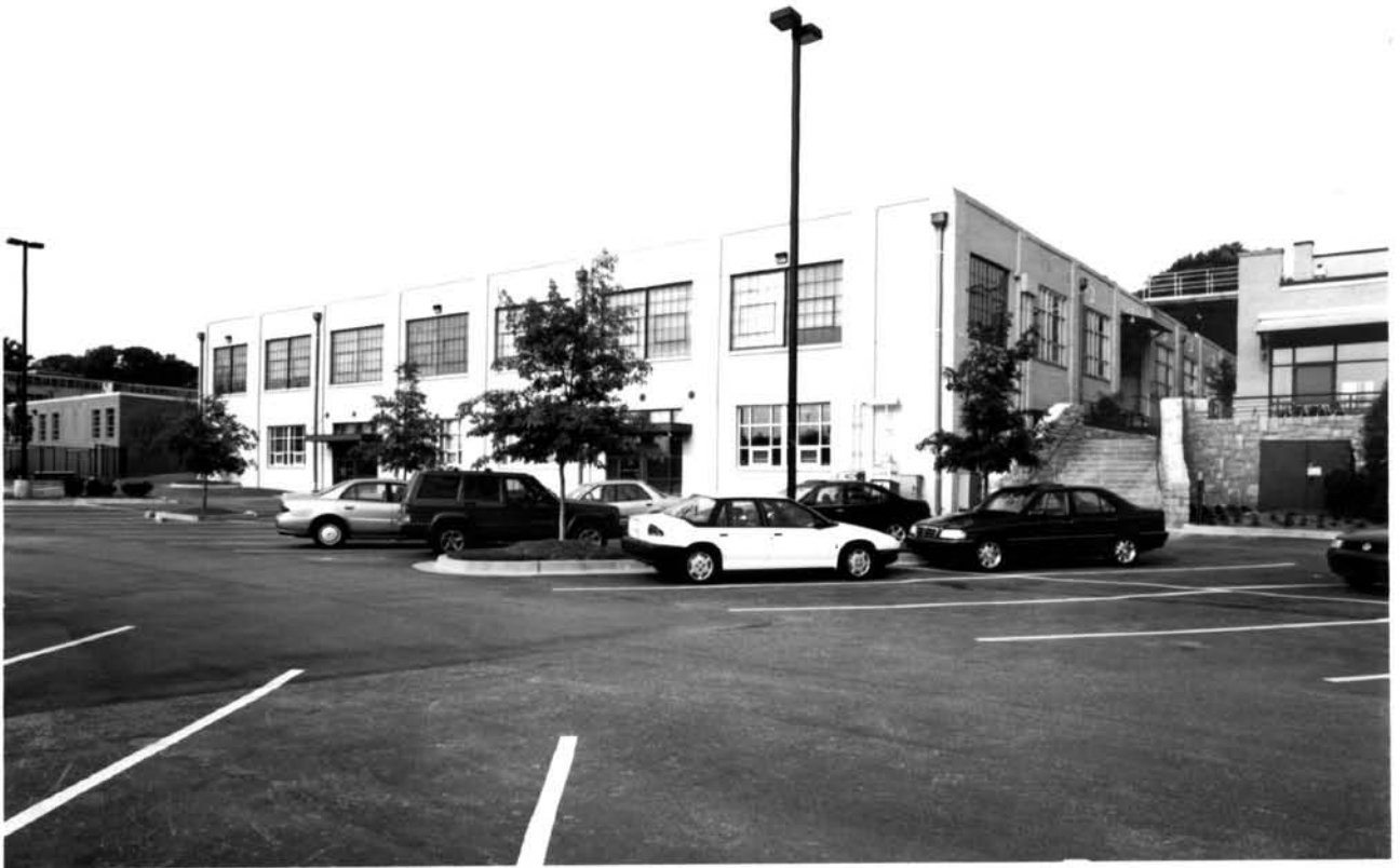
EMPIRE MANUFACTURING COMPANY BUILDING ATLANTA, FULTON COUNTY, GEORGIA PHOTOGRAPH 4 OF 15
