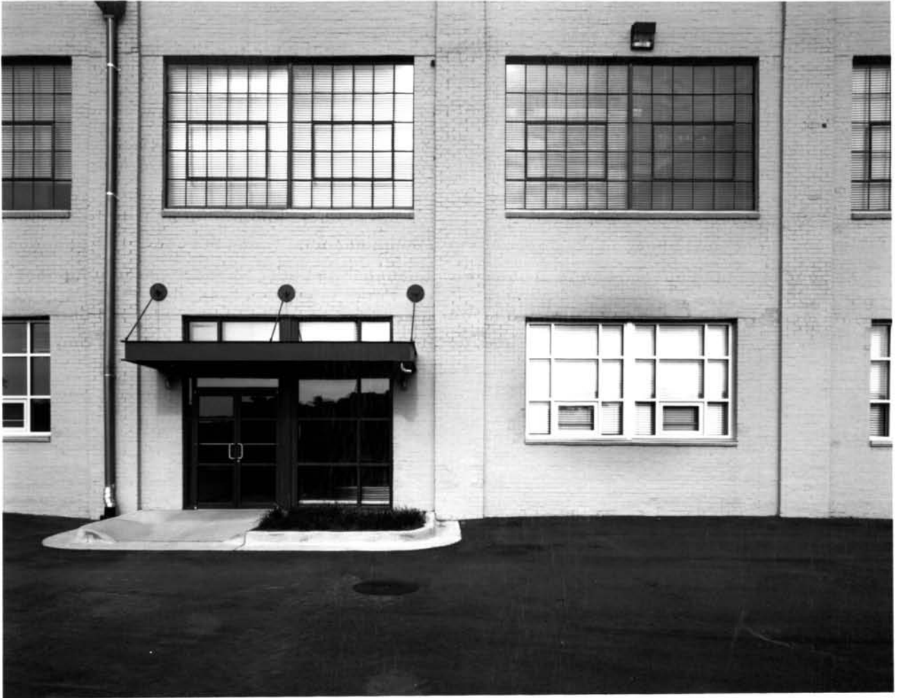
EMPIRE MANUFACTURING COMPANY BUILDING ATLANTA, FULTON COUNTY, GEORGIA PHOTOGRAPH 13 OF 15
