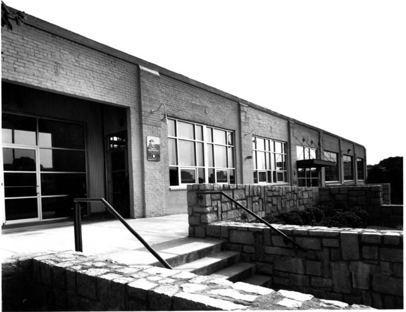
EMPIRE MANUFACTURING COMPANY BUILDING ATLANTA, FULTON COUNTY, GEORGIA PHOTOGRAPH 7 OF 15
