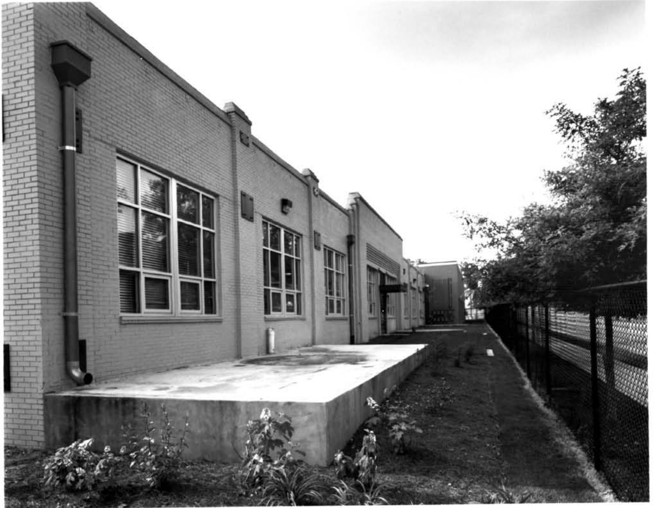
EMPIRE MANUFACTURING COMPANY BUILDING ATLANTA, FULTON COUNTY, GEORGIA PHOTOGRAPH 2 OF 15
