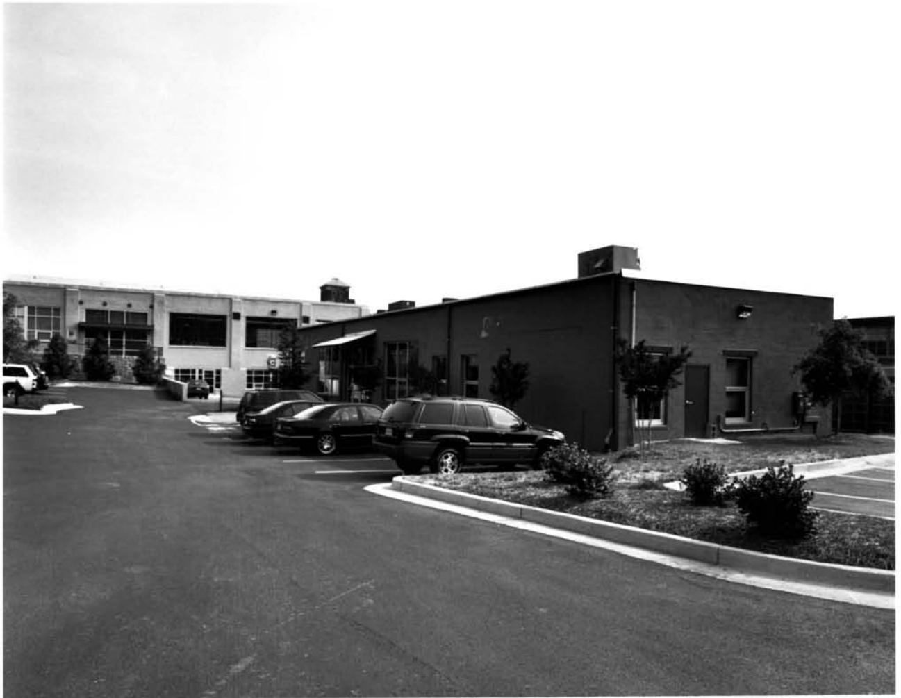
EMPIRE MANUFACTURING COMPANY BUILDING ATLANTA, FULTON COUNTY, GEORGIA PHOTOGRAPH 10 OF 15
