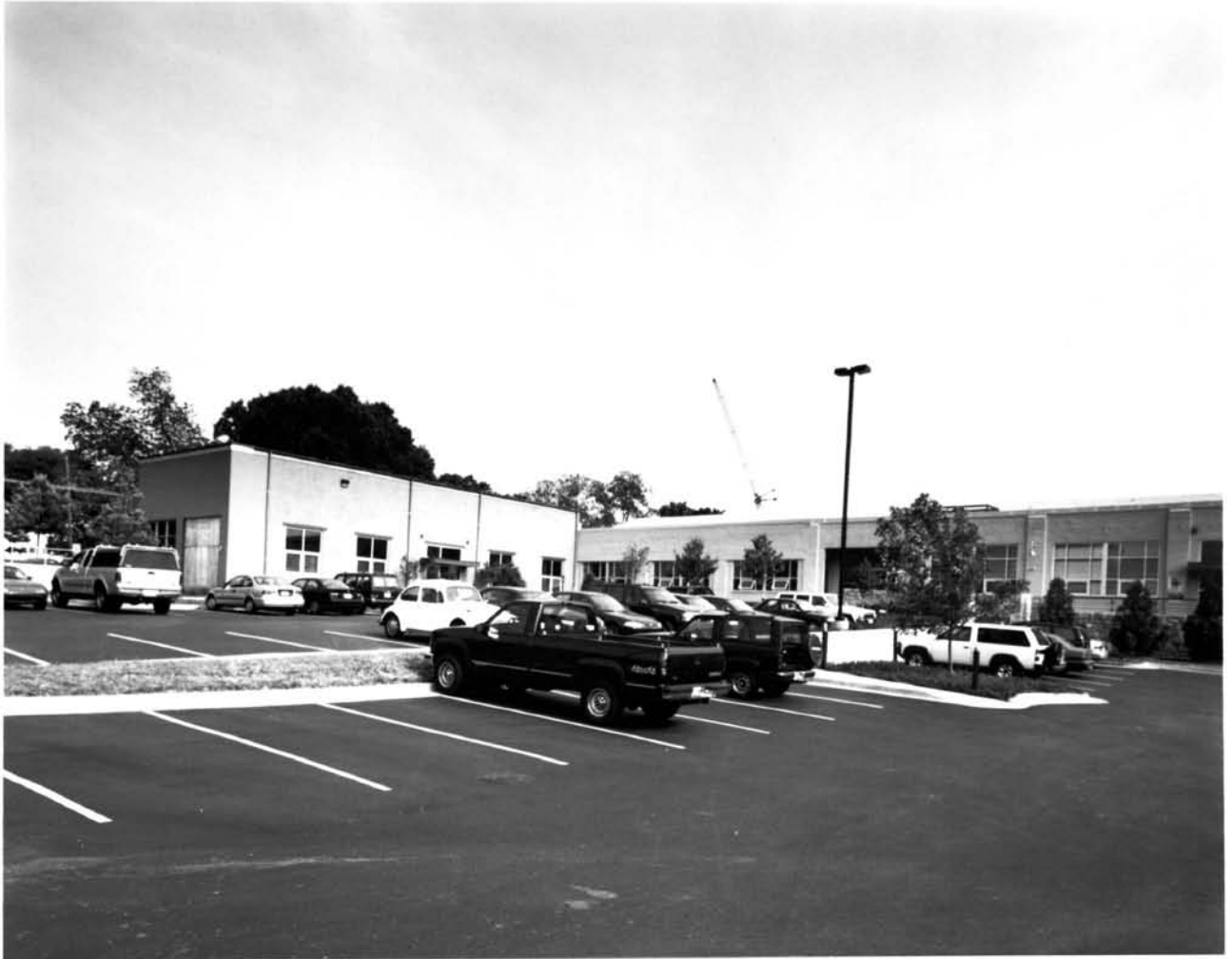
EMPIRE MANUFACTURING COMPANY BUILDING ATLANTA, FULTON COUNTY, GEORGIA PHOTOGRAPH 8 OF 15
