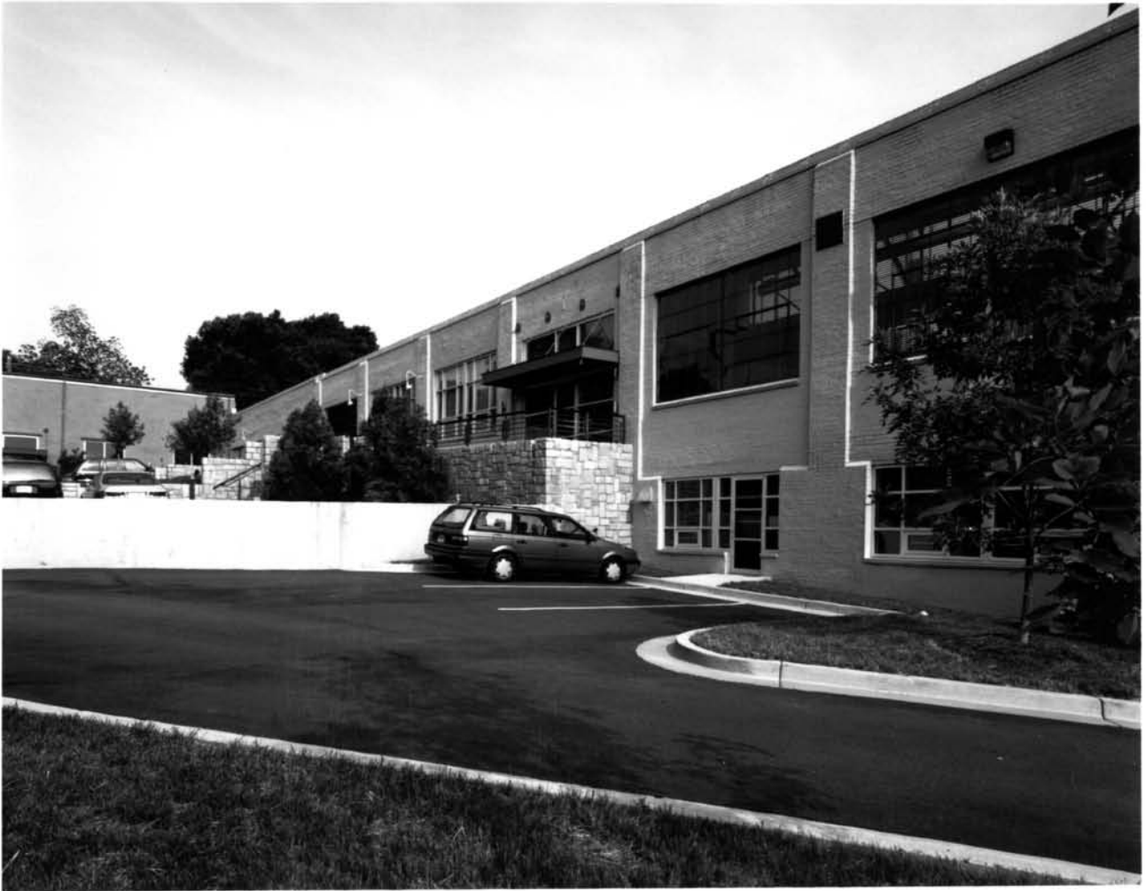
EMPIRE MANUFACTURING COMPANY BUILDING ATLANTA, FULTON COUNTY, GEORGIA PHOTOGRAPH 9 OF 15
