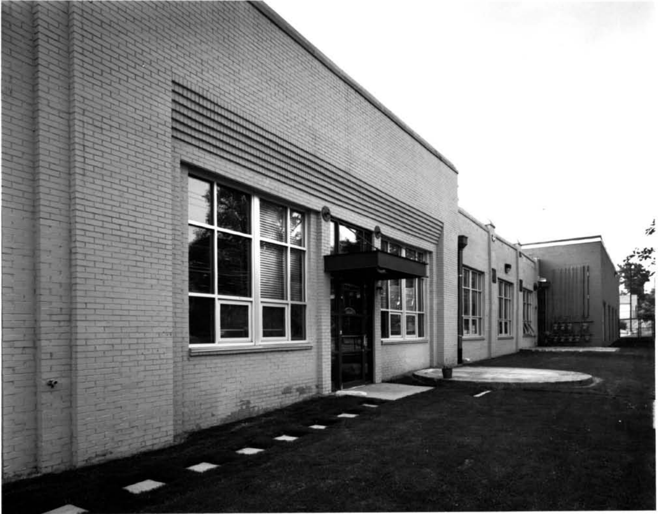
EMPIRE MANUFACTURING COMPANY BUILDING ATLANTA, FULTON COUNTY, GEORGIA. PHOTOGRAPH 1 OF 15
