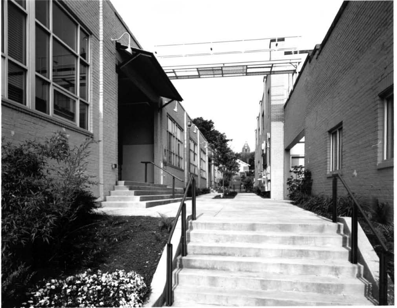
EMPIRE MANUFACTURING COMPANY BUILDING ATLANTA, FULTON COUNTY, GEORGIA PHOTOGRAPH 3 OF 15
