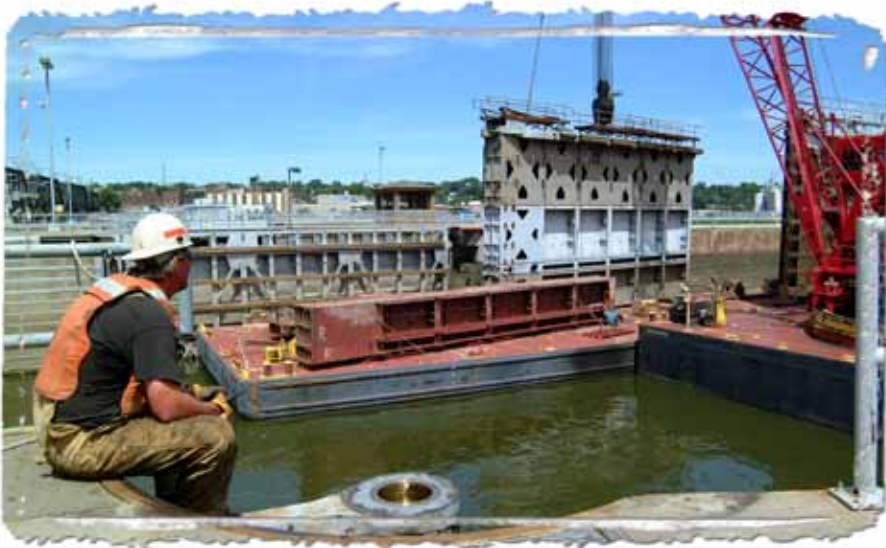
Below - Rodney Stover, Mississippi River Maintenance Crew, patiently waits while the Corps' largest crane, the Quad-Cities, is used to lift the first temporary miter gate off the barge from the Mississippi River Project Office.
