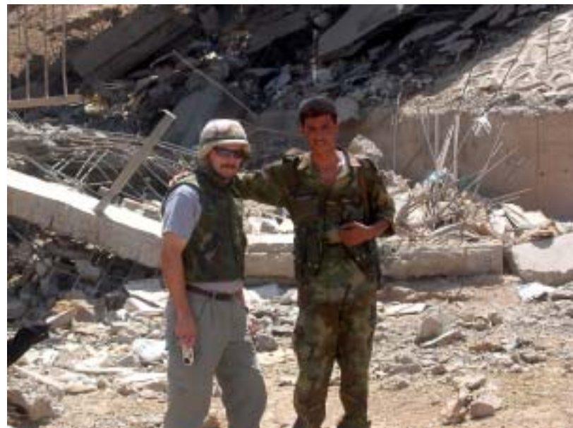
Mark Hoague, Engineering Division, stands next to an Iraqi Army soldier at a bridge site near Mosul in the northern region of Iraq. Hoague was on a field trip to understand the scope of repairs necessary to reopen the bridge.
