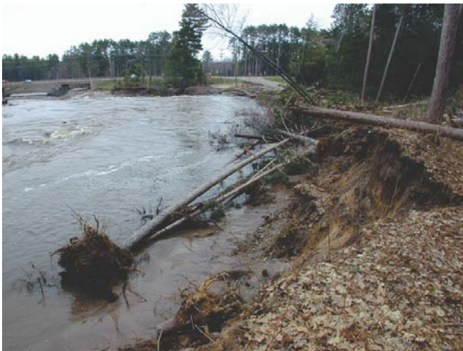
Before EWP recovery assistance: Tourist Park streambank erosion. (May 2003)
