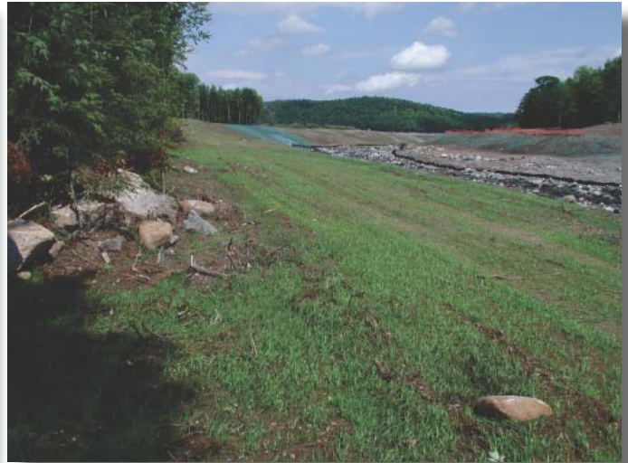
After EWP recovery assistance: Streambanks have been sloped and seeded. (July 2003)
