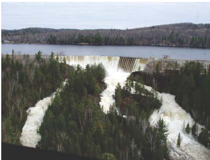
Downstream of the Silver Lake Basin, the Dead River Basin spillway overflowed during the flood.
