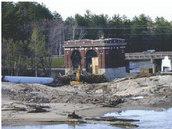
Debris removal at Tourist Park substation.
