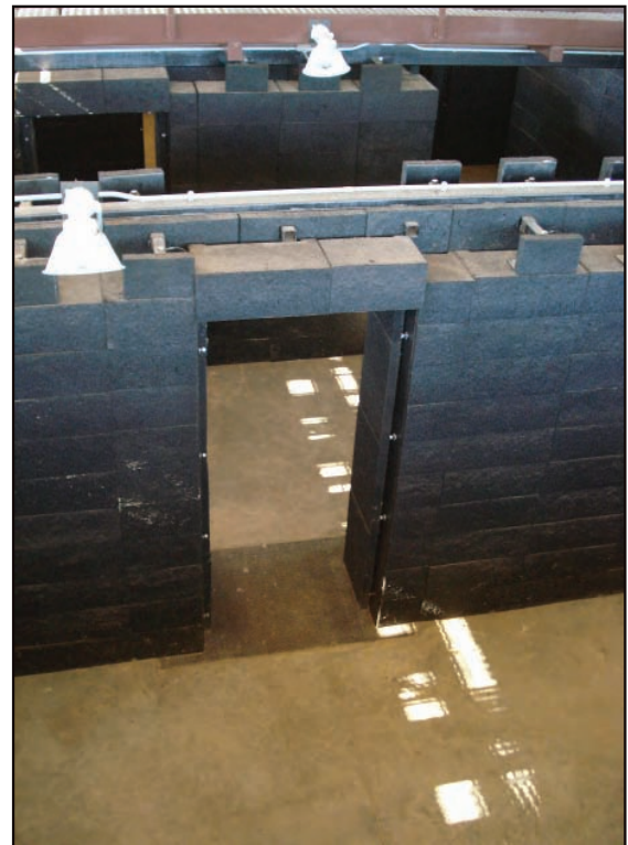
The top of the Shoothouse equipped with a catwalk to allow for observation while Soldiers are training.
