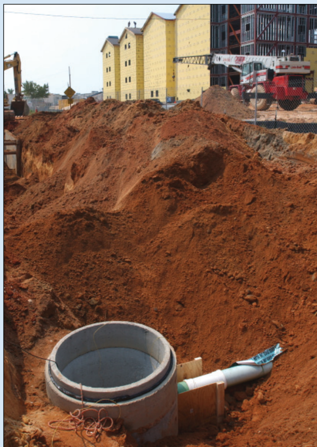
Contractors reroute infrastructure on Second Brigade Barracks at Fort Bragg.
