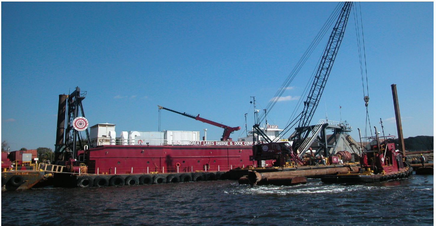
The Florida is getting ready for work at the Brunswick Harbor.
