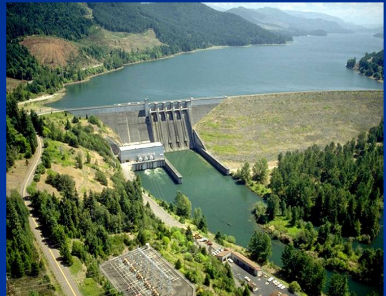
Lookout Point Dam
