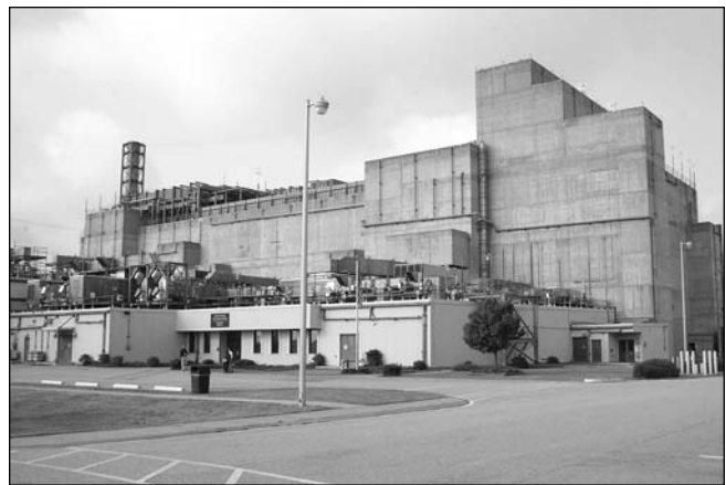
Exterior view of the Defense Waste Processing Facility
