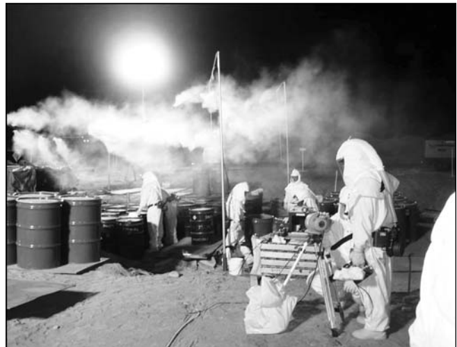
Waste characterization using misters
