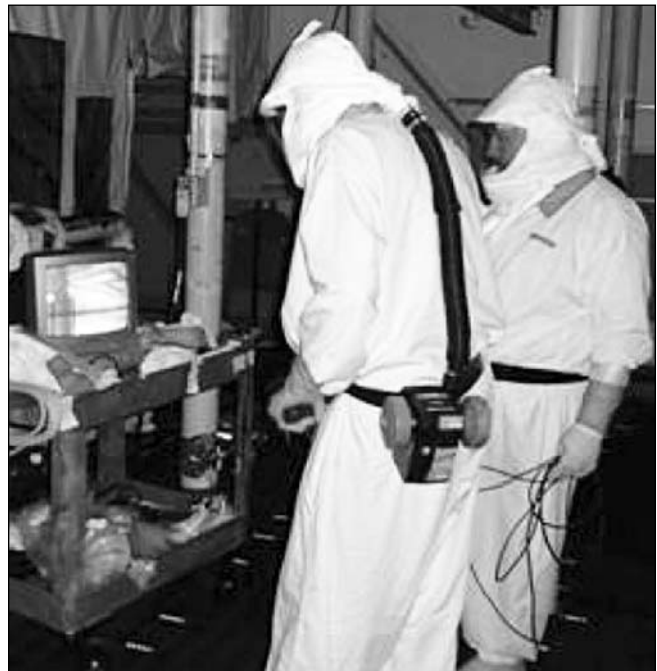
K Basin final pass vacuuming
