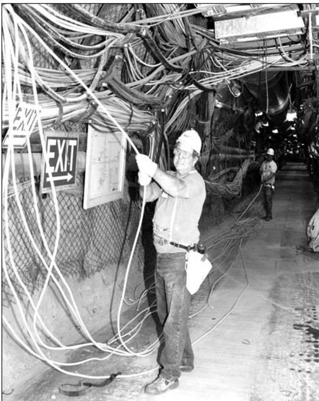
Legacy cable removal in U1a Complex (in-progress)
