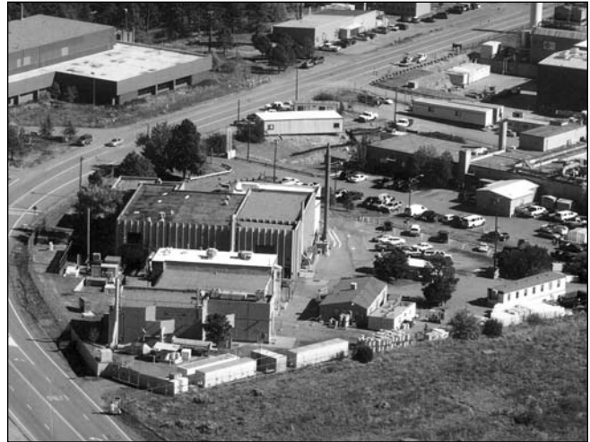
Waste Characterization, Reduction and Repackaging Facility, Los Alamos National Laboratory
