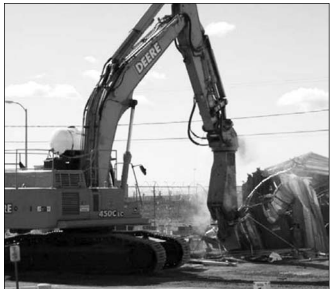
Demolition of 241Z
