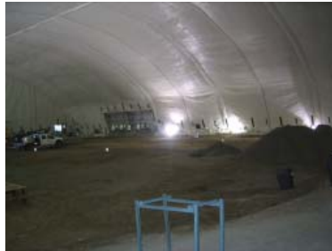
Accelerated Retrieval Project 2 Construction
