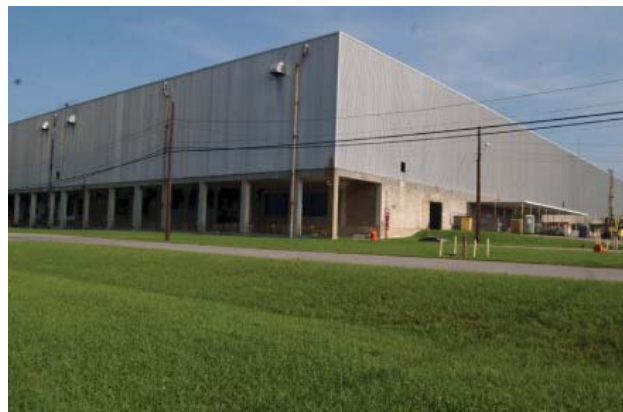
Southeast Corner of the K-29 Building
