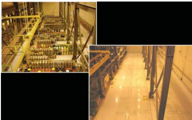
7725 Space Waste Cleanout To Remove Risk at Portsmouth
