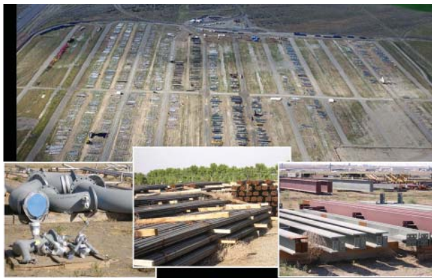
WTP Marshalling Yard
