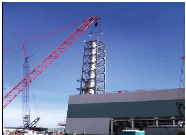
Setting of Low Activity Waste Facility Stack
