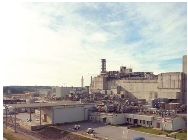
Defense Waste Processing Facility
