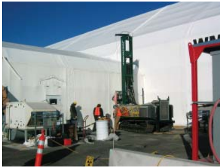
Accelerated Retrieval Project Foundation Stabilization
