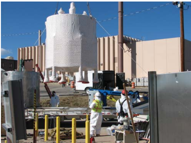
Workers Remove the 20+ Year-Old Caustic Tank at TA-50 Rad Liquid Waste Treatment Facility
