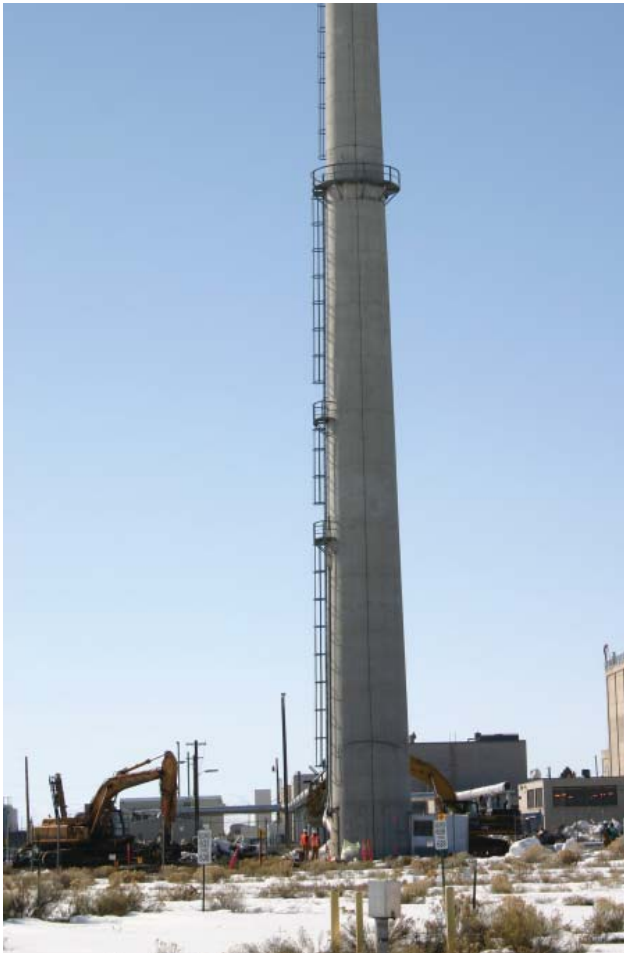
Preparations to Demolish the Engineering Test Reactor Stack
