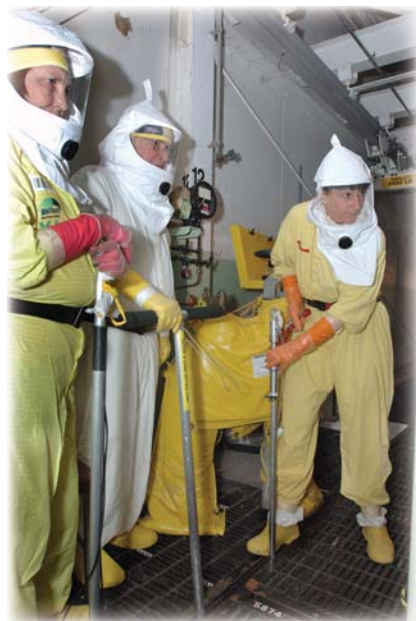
Consolidated Radioactive Sludge (an Estimated 55 Cubic Yards) Vacuumed from the Floors of Hanford's K East Basin. Began Transferring the Sludge Out of the Basin in Preparation For Draining and Removing the Leak-Prone Pool
