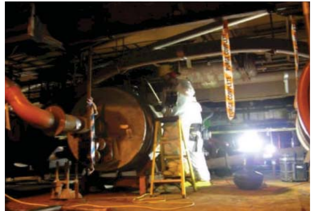
Vent/Purge/Drain Activities in K-25 Building
