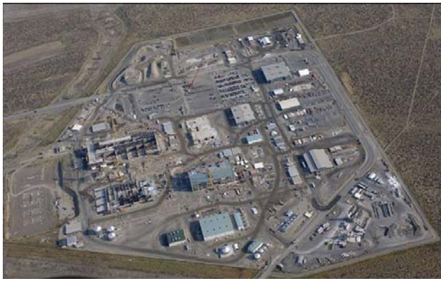
Aerial View of WTP Site
