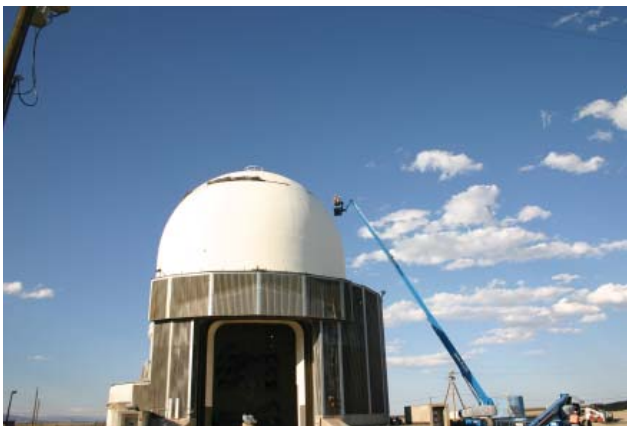
Crew Preparing To Demolish the Loss of Fluid Test Reactor Facility
