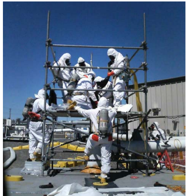
Replacing an In-Tank Video Camera in Tank C-103 To Support Waste Retrieval Activities
