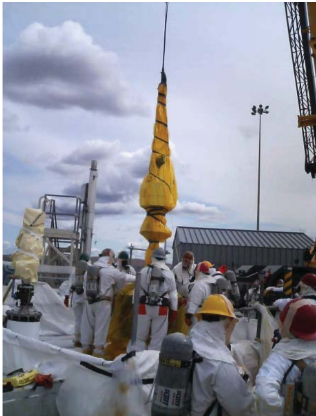
Removing a Failed Slucicer at Tank C-103
