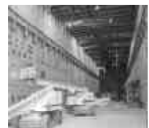
PRETREATMENT FACILITY HOT CELL AT THE OFFICE OF RIVER PROTECTION
