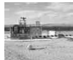
A NEW SLUDGE TRANSFER LINE AT K-EAST BASIN
