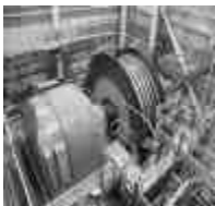
ANOTHER VIEW OF THE WASTE HOIST DRUM AND MOTOR AT THE WASTE ISOLATION PILOT PLANT.
