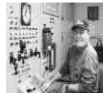
THE WASTE HOIST CONTROL ROOM AT THE WASTE ISOLATION PILOT PLANT.
