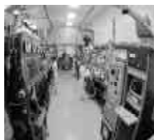
LOS ALAMOS NATIONAL LABORATORY PLUTONIUM FACILITY
