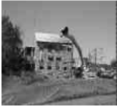
DEMOLITION OF THE 1940's/1950's ERA BUILDING AT Y-12.
