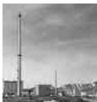
ENGINEERING TEST REACTOR STACK DEMOLITION AT THE REACTOR TECHNOLOGY COMPLEX.
