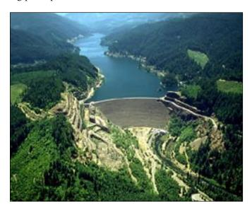
Cougar Lake has a storage capacity of 219,000 acre-feet and controls runoff from an area of 208 square miles. The lake's surface area is 1,235 acres at full pool. The dam rises 445 feet above the streambed.
