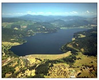
Dorena Dam controls the Row River and reduces flood stages downstream on the Willamette. Dorena Dam is a 145-foot-high earthfill and concrete structure with spillway and outlet works near the right abutment. Authorized primary project purposes are flood control, navigation improvement, and irrigation. Repairs to 560 linear feet of the Jenkins Location revetment, part of the Dorena Dam project, were undertaken in 1998 to repair damages caused by flooding in 1996.
