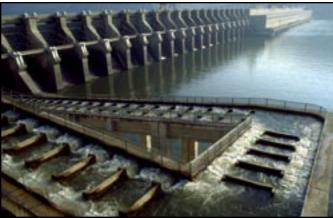
Mitigation Program, contracts were awarded in 1996 for a new fish passage system and flow deflectors. The fish passage system will include a 1,200-foot-long, five-foot-wide, 20-foot-deep chute extending along the Oregon shore from the powerhouse to the dewatering building. From the dewatering building, the young fish will travel through a three-foot-diameter flume to the sampling and monitoring building. After being monitored, the fish will be returned to the river downstream of the power-
