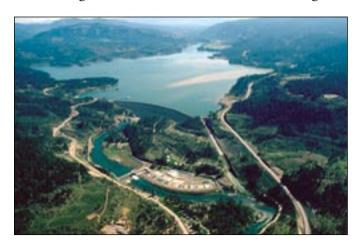
lating outlet tunnel, power penstock, and intake tower with multi-level intakes are located in the dam's right abutment; a gate-controlled concrete chute spillway is located in the left abutment. The powerhouse has a generating capacity of 49,000 kilowatts.
