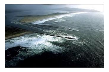
The 5,700-foot-long north jetty was constructed in 1933, rehabilitated in 1965, and again in 1991. In 1965, construction of a south jetty 8,000 feet long was authorized. Work began in 1969 and the first segment was finished in 1971. Construction of the second segment was completed in 1974. Construction of the third segment— 1,500 feet to complete the 8,000-foot jetty—started in 1978 and was completed in 1979.
