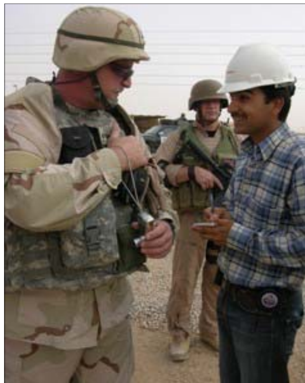
Mike Miller (left) talks with his Iraqi contractor at the job site of the Baghdad Police Academy (North) in Mosul. Miller said although the project is massive, the contractor makes progress every week; he is safety-conscious; and his quality work is immediately obvious. [USACE Photo by LuAnne Fantasia]
