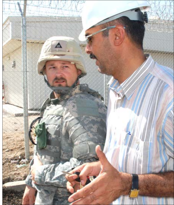
USACE Project Manager Jim Marple checks construction quality at the new $28.8 million prison being built near Nasiriyah in southern Iraq. (USACE photo by Norris Jones)
