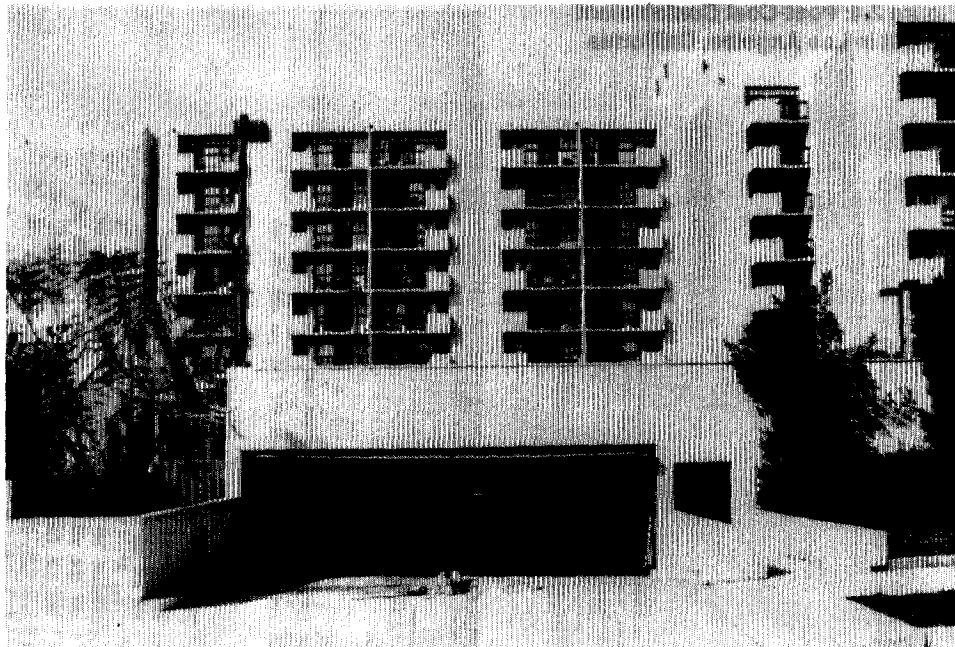
Figure 2.3: Precast Containment Project in Los Angeles, California
