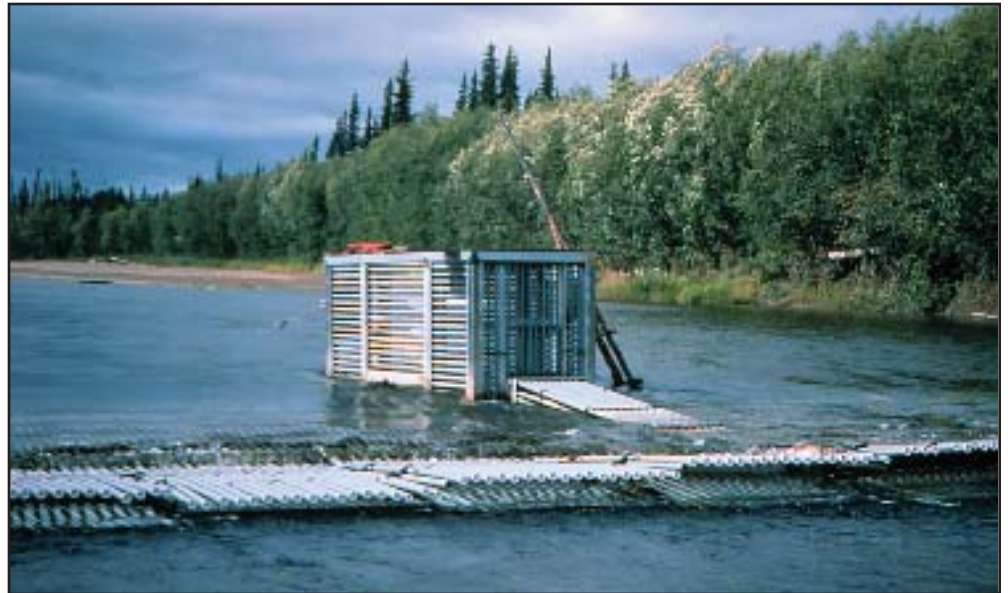
Resistance board weirs like this one are an important tool to determine salmon run timing and total numbers of spawning fish.
