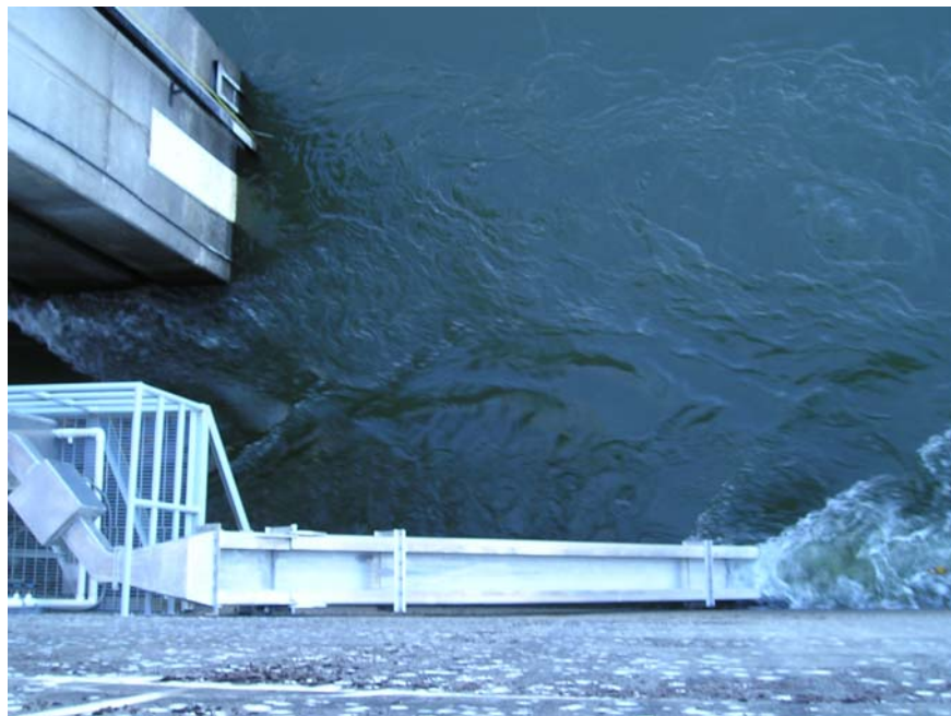
Figure 2. Lamprey collector at the Washington-shore downstream fishway entrance.
