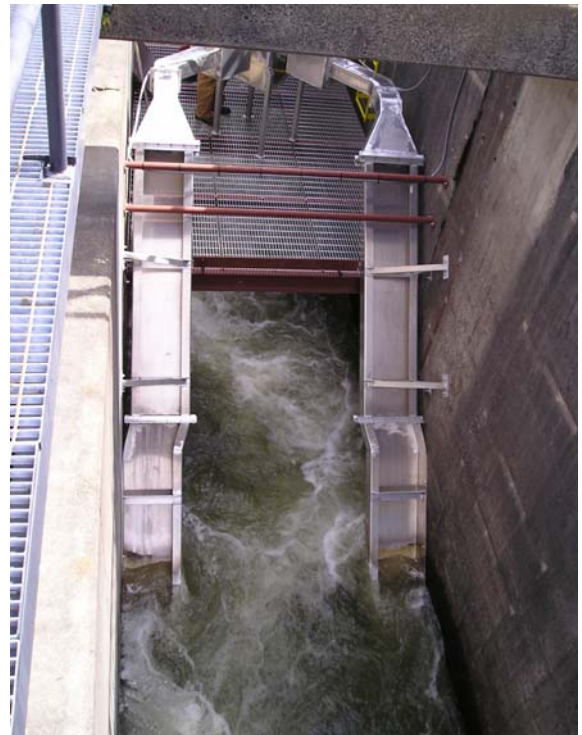
Figure 2. Prototype lamprey collectors tested in the Bradford Island AWS.
