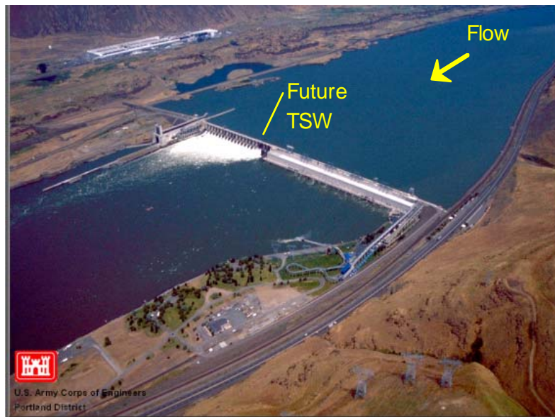
Figure 1. Aerial Photograph of John Day Dam Showing the Location of the Future Top Spill Weirs (TSW).
