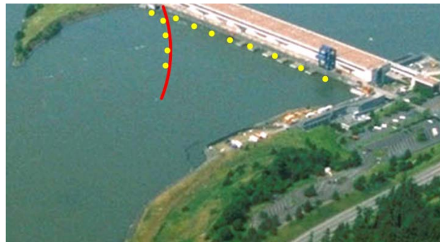
Figure 3. Photograph Showing Proposed Locations (yellow dots) of Cabled Hydrophones. All locations on the face of the dam will would have one deep hydrophone near elevation 30 ft above mean sea level (MSL) and one shallow hydrophone near elevation 68 ft above MSL. Forebay locations will have single hydrophones attached to the BGS and facing upstream
