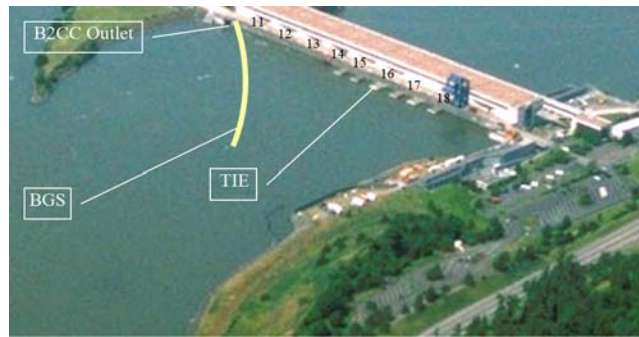
Figure 1. Photo of the B2 forebay showing the B2CC surface flow outlet, turbines 11-14 without turbine intake extensions (TIES), and turbines 15-18 with TIES. The yellow curved line represents the likely location of a 400-ft long BGS upstream of turbines 11-14. The BGS will be anchored to the Washington shore on the upstream end and just to the north of the B2CC outlet on the downstream end.
