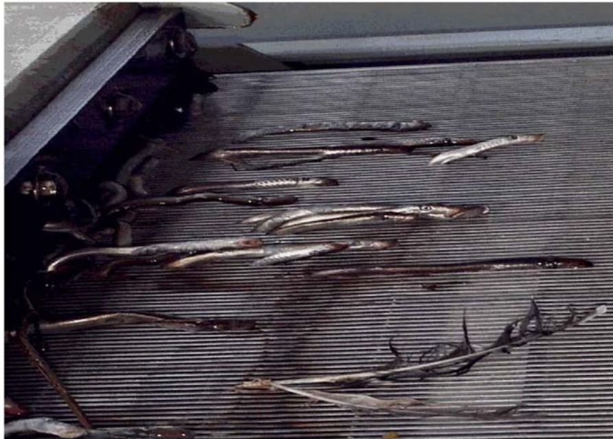
Figure 2. Pacific lamprey macrophthemia impinged on screens at the John Day Juvenile Bypass System. Photo courtesy of the Columbia River Intertribal Fish Commission.
