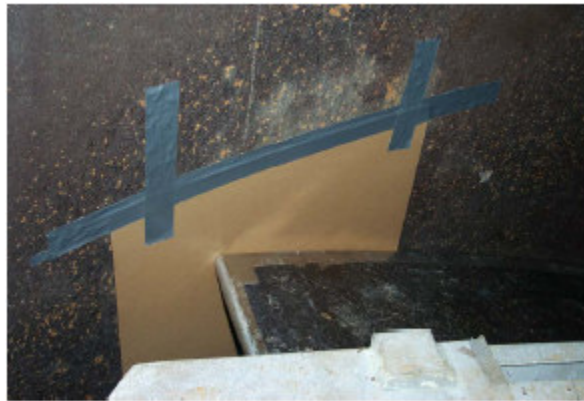
Figure A - 18. Example of tracing runner blade on discharge ring
