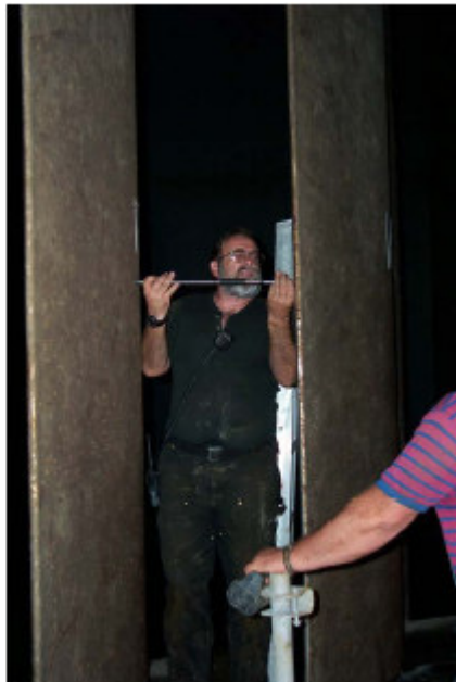
Figure A - 22. Example of measuring the wicket gate opening
