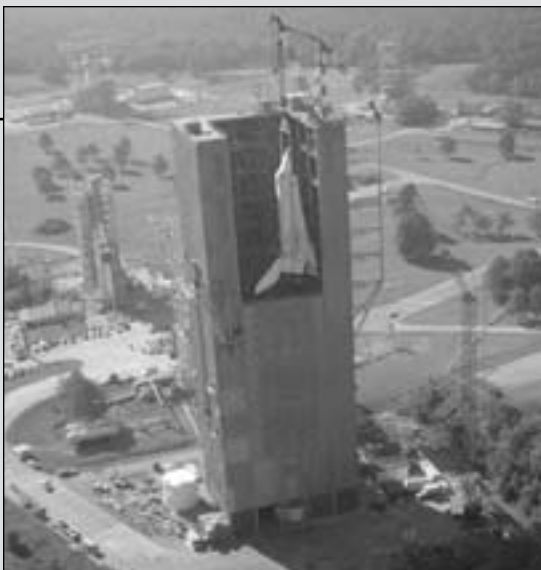
Space Shuttle Enterprise is lifted into the Dynamic Test Stand. (7992403)
