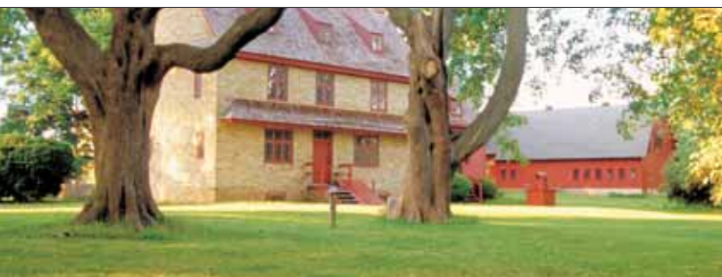
Left: The ruins of Sheldon Church in Beaufort County, South Carolina, burned by the British in 1779, rebuilt, and burned again by General Sherman during the Civil War. Below: The William Brinton House, a national historic landmark, survived the Battle of Brandywine.
