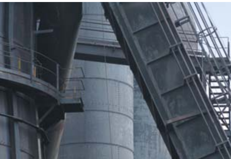
Above and right: Views of the Carrie Furnace complex, once a key cog in the U.S. Steel empire, now silent. Rivers of Steel National Heritage Area hopes to convert the complex into a museum.
