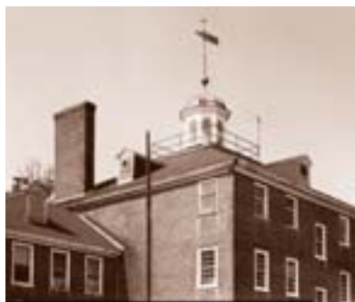
Far left: HABS architectural historians Jamie Jacobs and Catherine LaVoie documenting the quarantine station. Near left: The cupola offered a vantage point to see ships with immigrants approaching.
