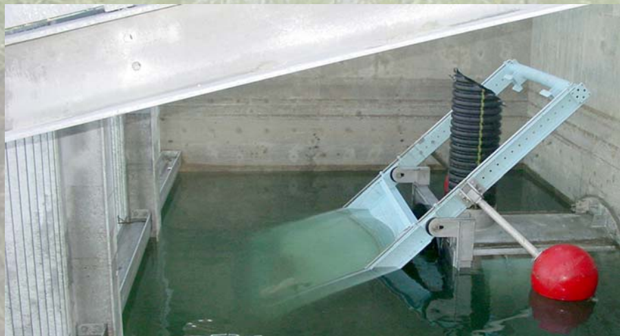
A flapgate—the simple thing that made the wetlands a reality.
