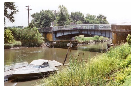
BRIDGE OVER OLD BRANCH CANAL - DEL. CITY
