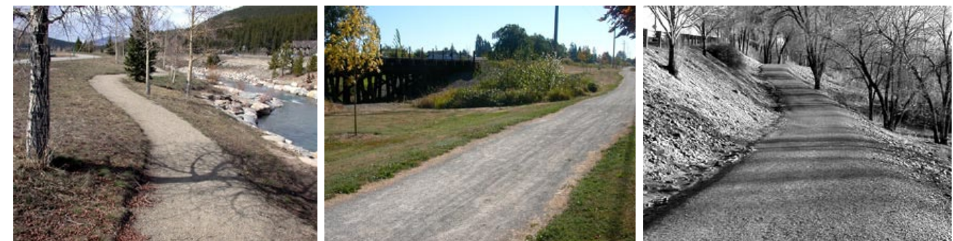
PHOTOS OF TYPICAL MULTI-USE TRAILS CONSTRUCTED WITH STONE FINES
