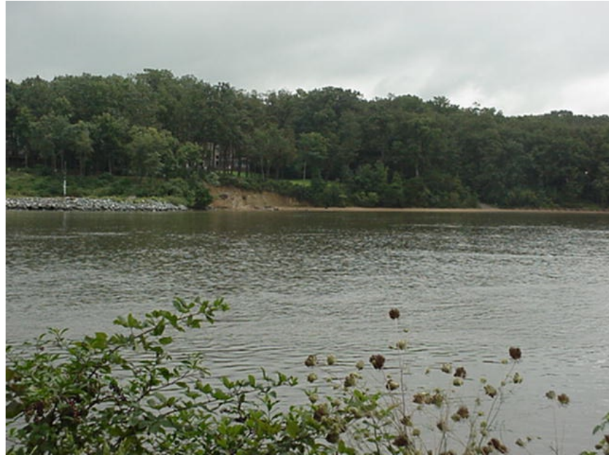
PHOTO 14. STATION 83+200, SOUTH SIDE, 30 AUG 04. LOOKING AT THE SLOUGHING FROM THE NORTH SIDE OF THE CANAL.
