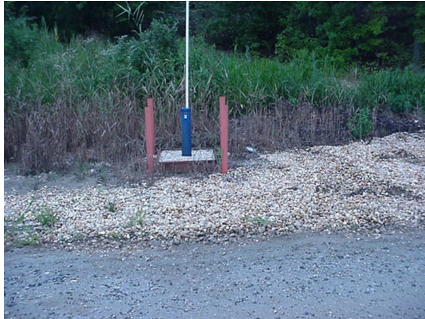
PHOTO 8. STATION 54+900, NORTH SIDE, 30 AUG 04. INCLINOMETER INSTALLED TO MONITOR SLOPE MOVEMENT.
