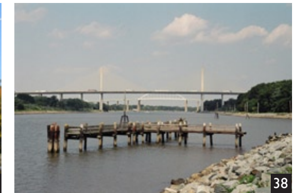
VIEW TO S.R. I BRIDGE
