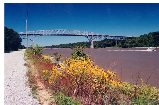
SUMMIT BRIDGE - DELAWARE
