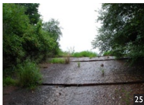
GUTHRIE RUN DRAINAGE CULVERT
