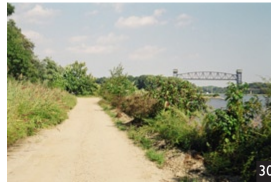
SERVICE ROAD ADJACENT TO DEEP CUT
