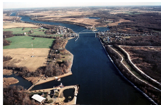
C&D CANAL - CHESAPEAKE CITY BRIDGE - (LOOKING EAST)
