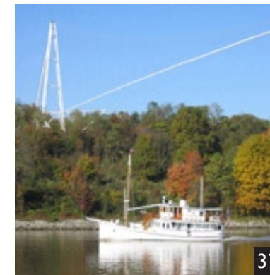
UTILITY SPAN EAST OF RR BRIDGE
