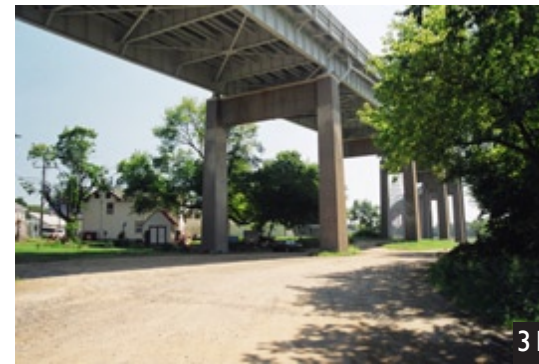
ST. GEORGES BRIDGE NORTH
