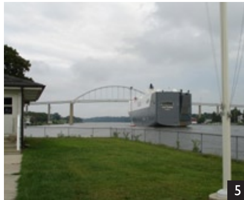
USACE FIELD OFFICE OVERLOOKING CANAL
