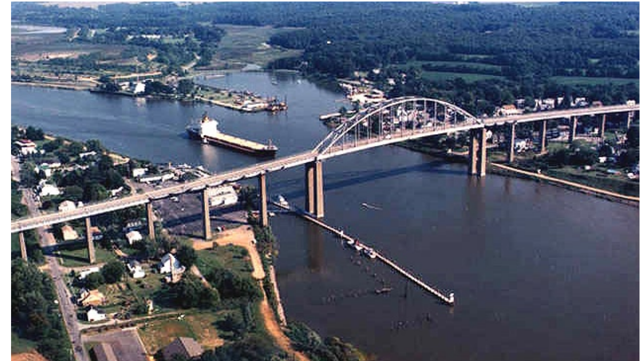
3. C & D CANAL AT CHESAPEAKE CITY, MARYLAND. MD-213 CROSSES THE 2-LANE BRIDGE, WHICH HAS 135 FEET OF VERTICAL NAVIGATIONAL CLEARANCE ABOVE THE AVERAGE HIGH TIDE WATER LEVEL. PHOTO IMAGE COURTESY OF THE U.S. ARMY CORPS OF ENGINEERS.
