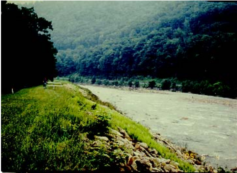
A levee/flood wall system was constructed along the North Branch of the Potomac River to prevent flooding at Kitzmiller, Garrett County, Maryland.
