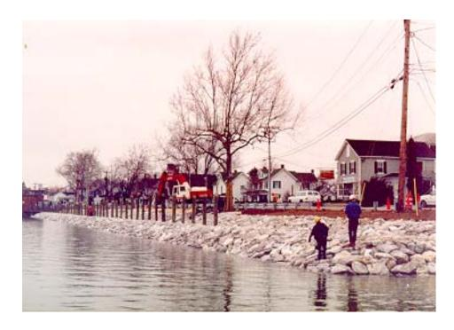
A stone revetment was constructed at Solomons Island, Calvert County, Maryland, to protect the roadway from further storm-induced erosion and potential structure failure.
