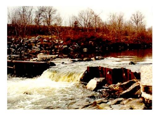
Flood control projects, such as this drop structure, are designed to reduce flood hazards by improving the flow rate of the stream. However, in this case, the vertical drop prevents fish from migrating upstream to spawn. The Corps will modify the structure to accommodate fish passage as part of the Section 1135 – Anacostia River Restoration Project.
