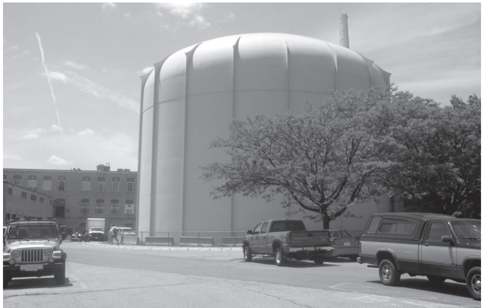
Figure 2: Research Reactor Building Surrounded by Jersey Barriers
