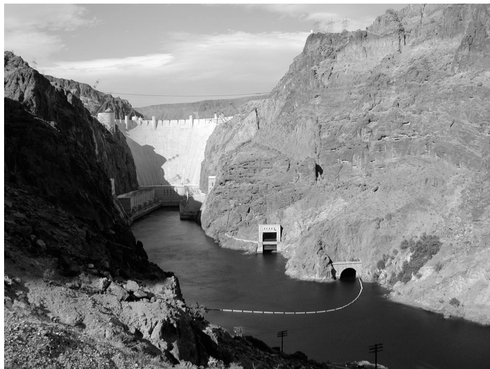
Figure 3: Hoover Dam and Linked Boom Line Used to Enhance Perimeter Security
