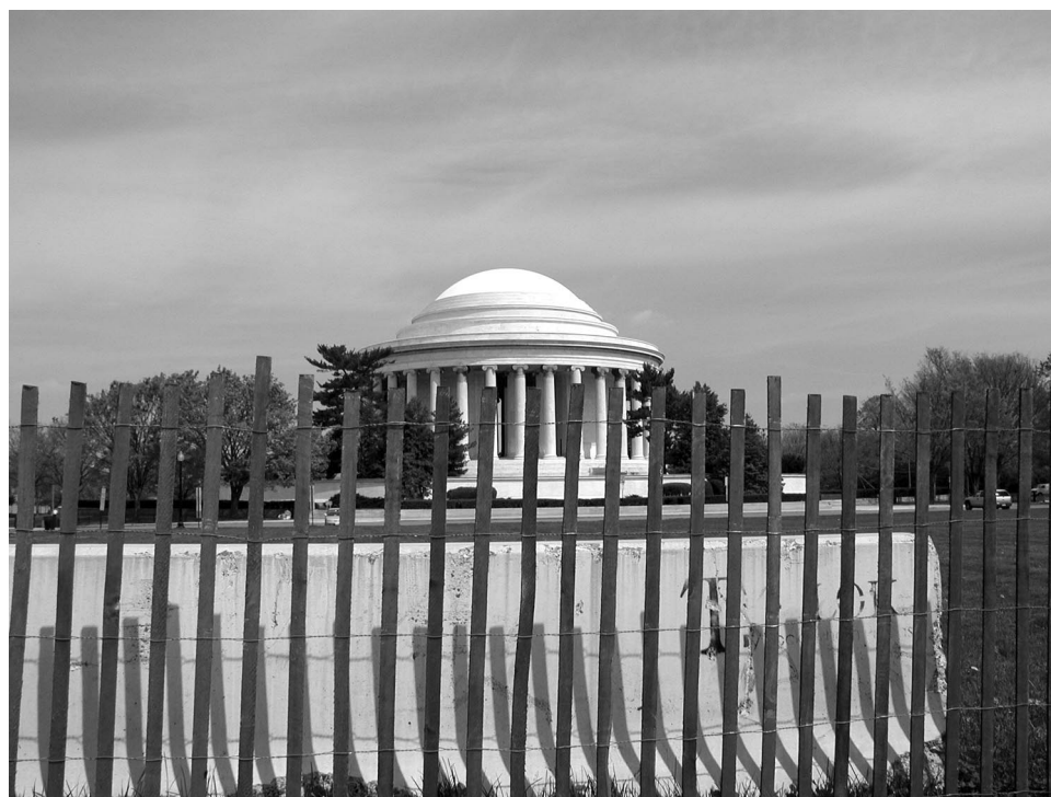
Figure 8: Jersey Barriers and Snow Fencing at the Jefferson Memorial
