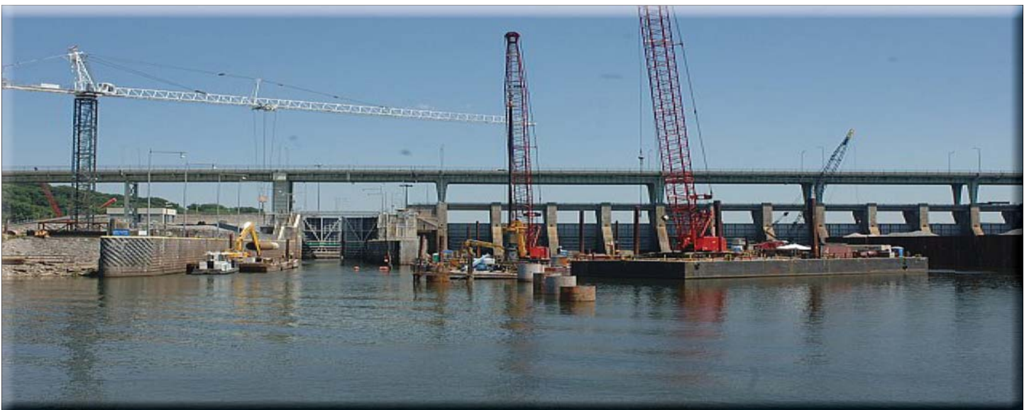
Tailwater construction of the cofferdam is underway at Chickamauga Lock.
