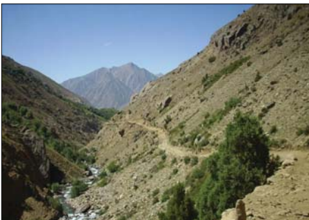
A narrow mountain road in Afghanistan needs widening for easier travel.
