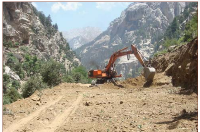
Bess’ team works in Afghanistan to widen a road.
