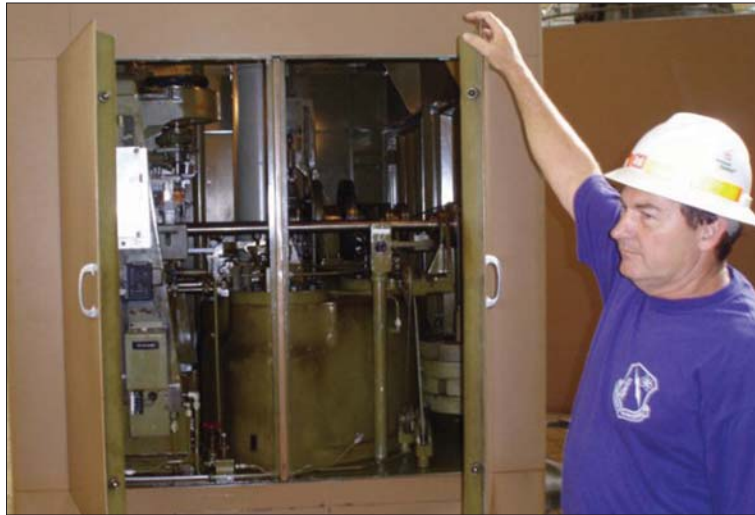
Senior Mechanic Jerry Kennedy explains the generator's governor function to the EAGLE Class.
