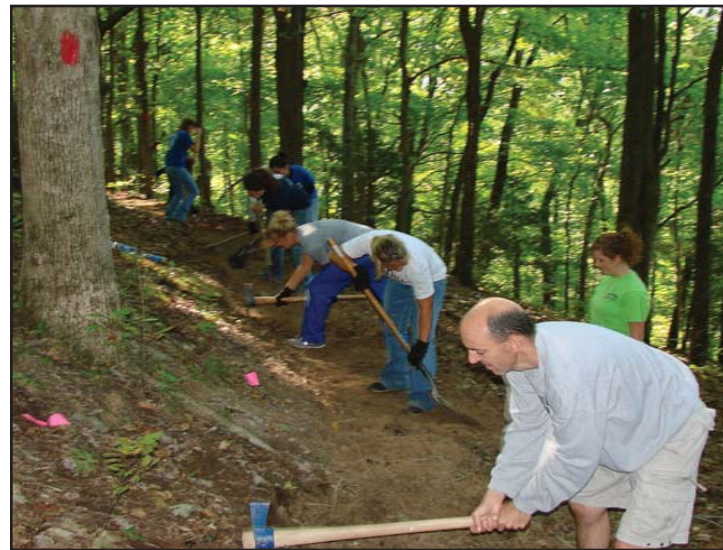
Volunteers construct a new section on the Bearwallow Gap Trail.
