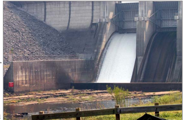
J. Percy Priest Dam spilling in 2005. The practice will add oxygen to the lower Stones River and improve the aquatic environment.
