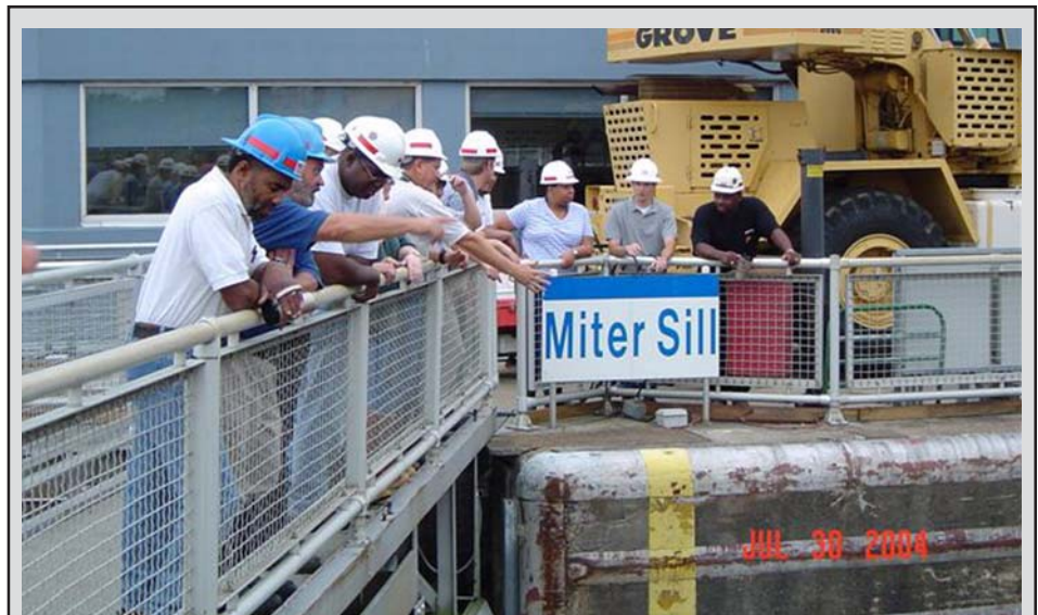
Members of the 2004 EAGLE class visited Chickamauga Lock July 30 and observed the lock dewatering process. Members now realize the tremendous amount of coordination that must take place between various Corps elements when a dewatering occurs. Project Manager Matt Tays met and escorted the class. Safety Specialist Bill Bennett helped answer questions posed by the group. Charlie Bryan explained the work performed by members of the Nashville District Dive Team around upstream intakes and the necessary safety measures that must be followed to perform such work. EAGLE team members descended into the empty lock chamber to view work up close. Most saw such areas for the first time. Several EAGLES even ventured inside the discharge ports to observe conditions visible only during dewatering.
