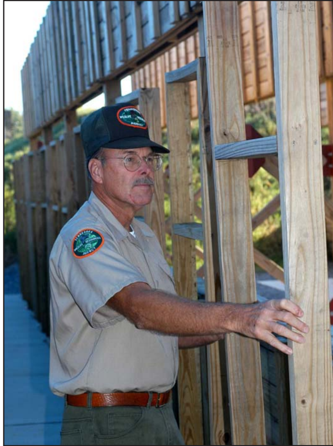
TWRA Shooting Range Manager Les Brown places a target holder in place on the new Stones River Shooting Range.
