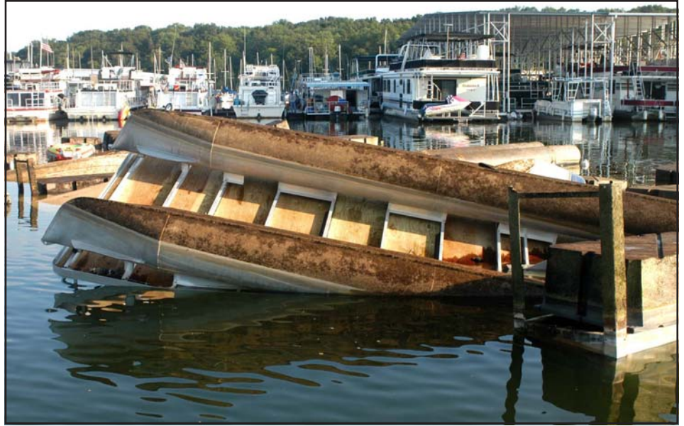
One of many overturned boats lies partially submerged Tuesday morning along what used to be “K” Dock at Elm Hill Marina before high winds flipped the structure.
