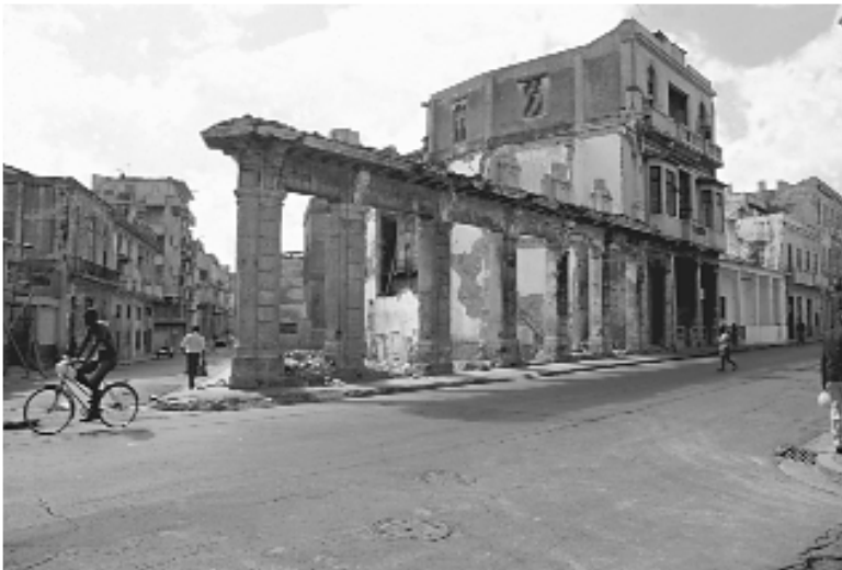
Remains of a collapsed building near the Malecon, Havana, Cuba. Photo by the author.
